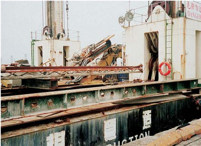
L-shaped plates were used to connect the sheet piles to the anchors
