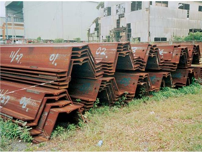
The deep excavation and seismic loads called for heavy-duty AZ 48 piles
