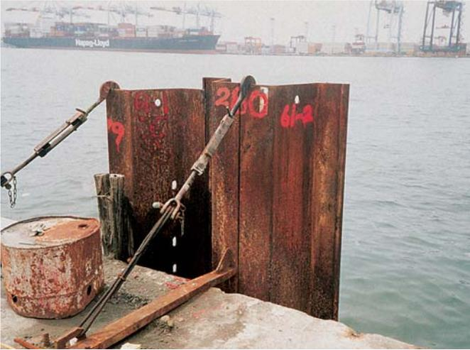
The piles were driven hard alongside the existing berths
