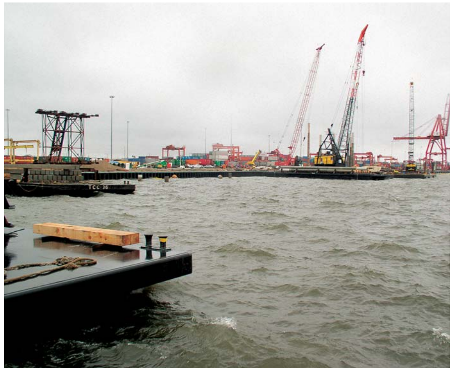
Overview of the construction site
