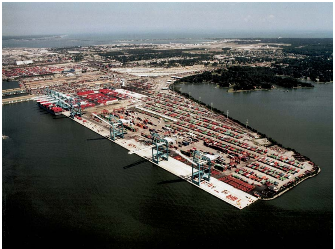
The NIT south wharf was renovated using two rows of steel sheet piles
