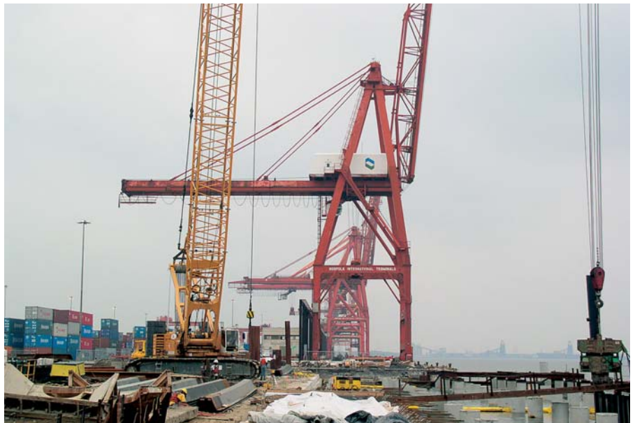
Installation by land-based crane equipped with vibratory hammer
