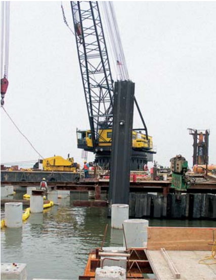
A template ensures the straightness of the sheet pile walls
