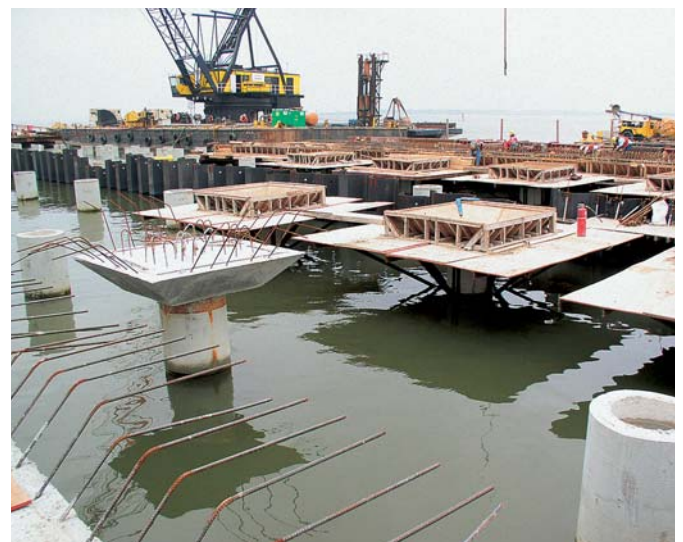
Supporting piles for the front side of NIT's new South Wharf
