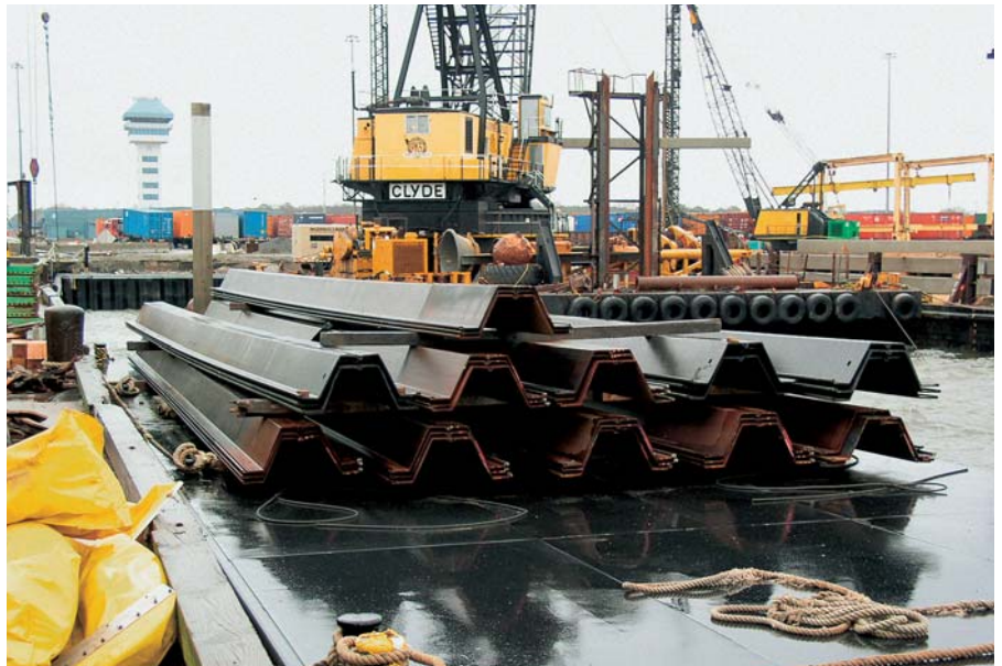
The AZ double piles were brought in by barge
