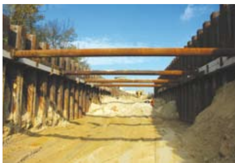
Construction phase of the underpass
