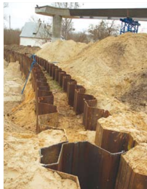
Steel sheet pile bridge abutment
