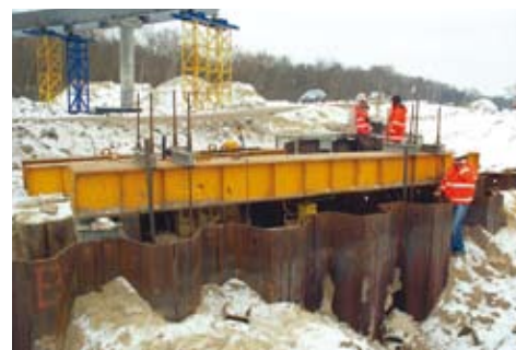
Static load test set-up
