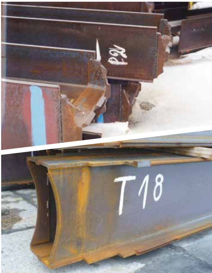
Fig. 17. Reinforcing of the tip of the pile with steel plates / shoes welded on the king pile toe.
