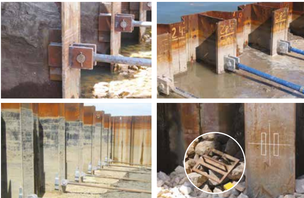
Fig. 5. Installation of the T-connectors at the job-site.
