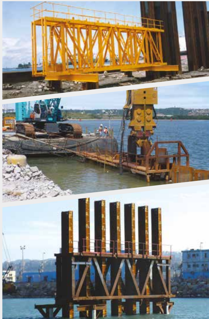
Fig. 9. Driving templates and their support.
