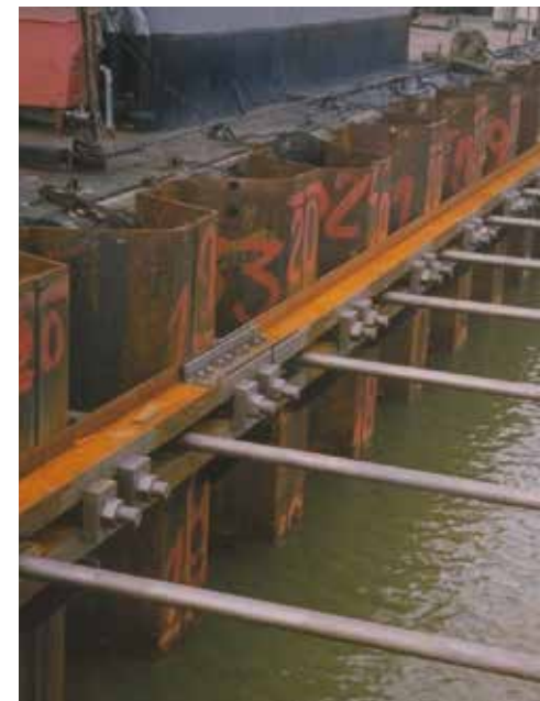
Fig. 6. Conventional anchor solution with tie-rods, walers,...
