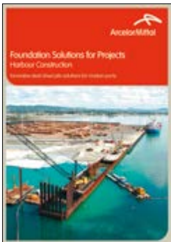
Harbour construction GB
