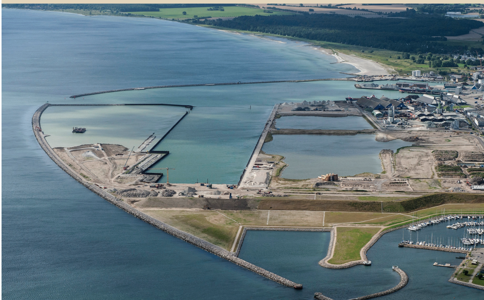
Aerial view during construction
