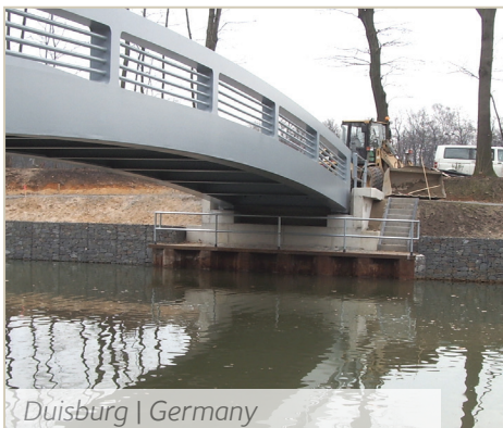
Temporary cofferdam | Germany
