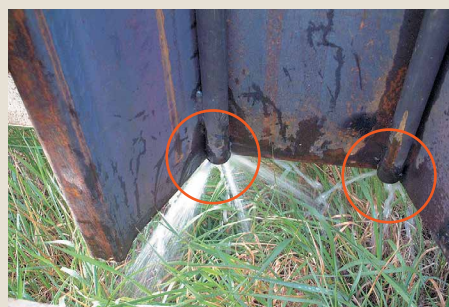
The jetting pipe ends flush with the toe of the sheet pile.
