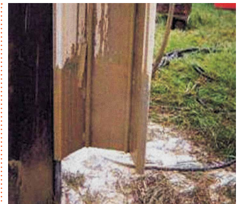
Photo 2 Extracting jetted U pile.
