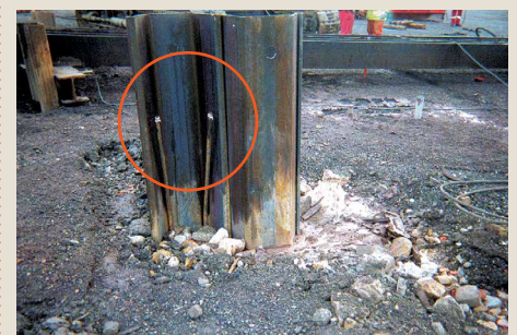
The top of the jetting pipe may be bent to facilitate connection of the supply hose.
