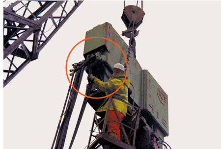
Hoses and jetting pipes being connected.
