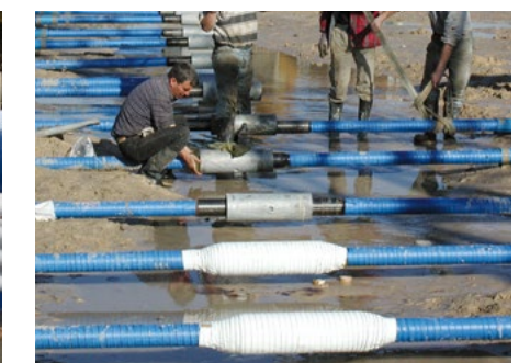
Site wrapping of connections
