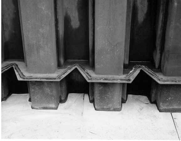
Fig. 2.1. Welded horizontal plates with hydrophilic strip.
