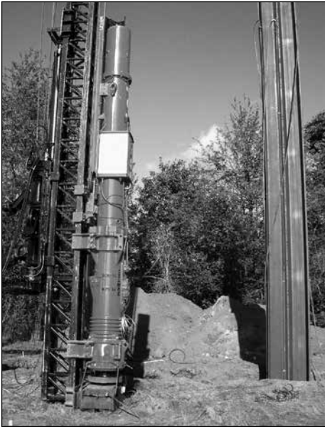
Fig. 11.6. Diesel hammer on fixed lead.
