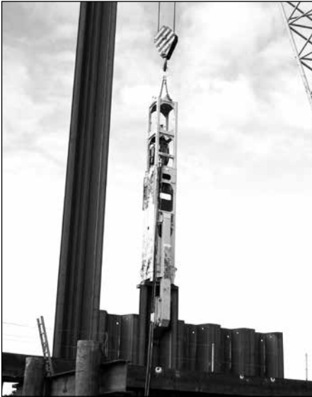
Fig. 11.8. BSP CX85 driving AZ piles.
