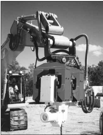
Fig. 11.14. Excavator mounted with vibratory hammer.
