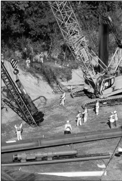
Fig. 11.7. Diesel hammer mounted on leader rig driving sheets.
