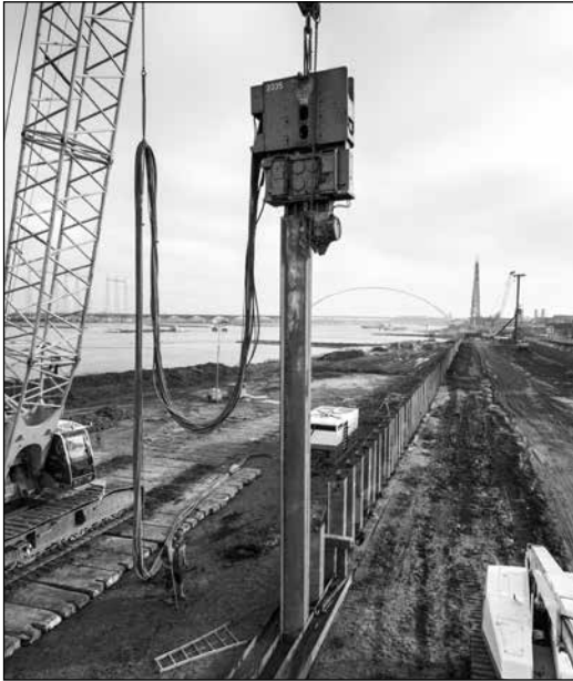
Fig. 11.2. Pitch and drive operation using guide walings at ground level to prevent excessive rotation of piles.
