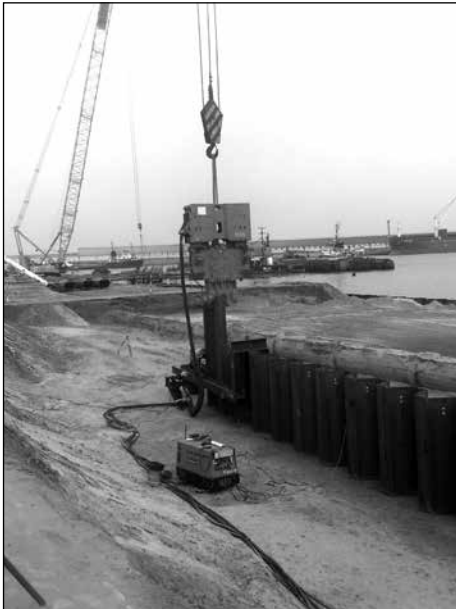
Fig. 11.10. Rope suspended HFVM vibratory hammer.
