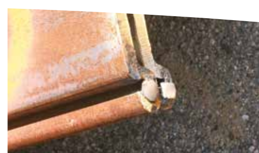
Bolt inserted in leading interlock.
