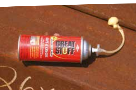
Closing interlocks with foam or grease.
