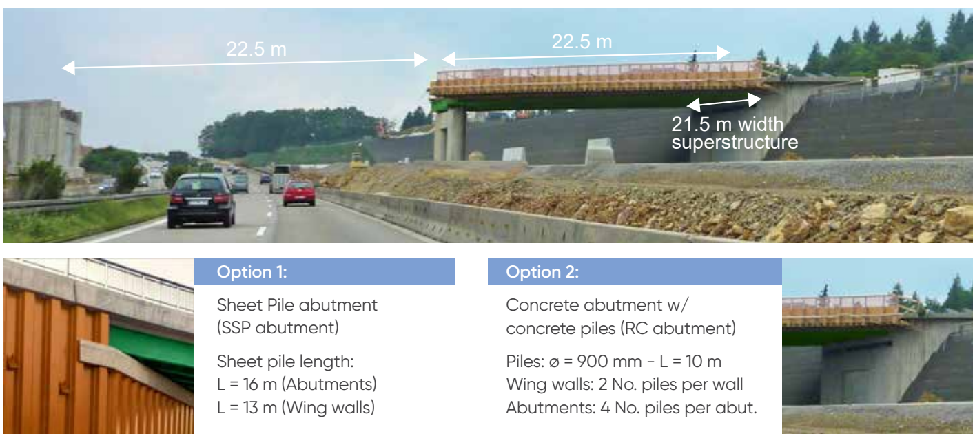
Fig. 7. Standard two-span bridge specification based on a real project: sheet pile abutment vs concrete abutment (ready-mix concrete).
