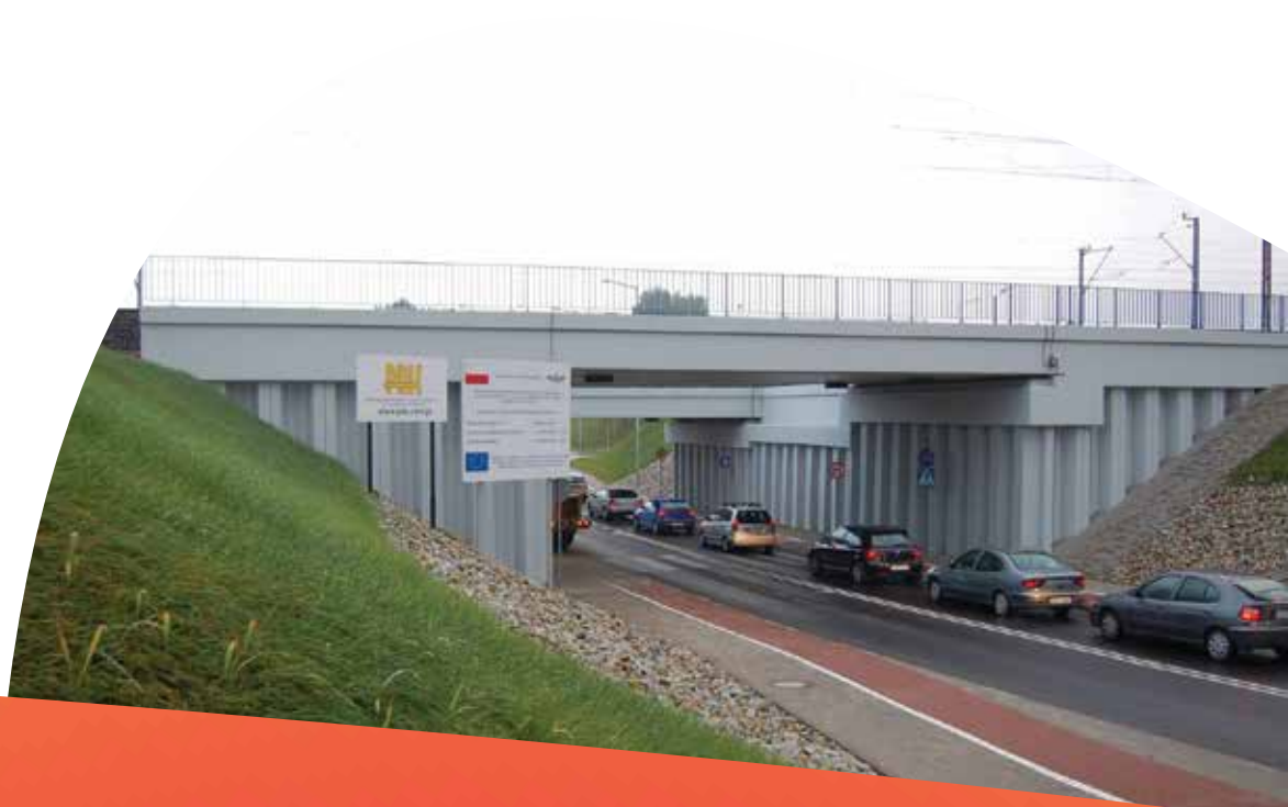
Fig. 1. Steel sheet pile (ca. 300 t of AZ 50) bridge abutment (Swarzędz, Poland).
