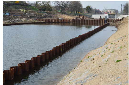
Fig 11 Wrocław – City Channel
