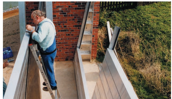
Raising of an embankment in Zons (Germany) – temporary closure of openings in the permanent flood defences
