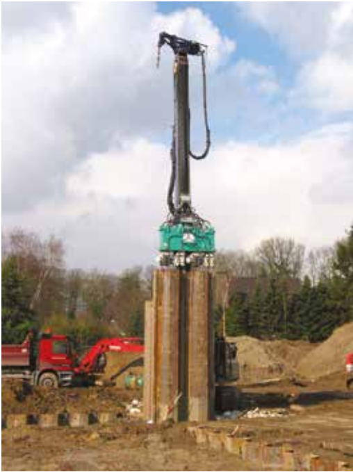
The sheet piles were installed with an ABI hydraulic press allowing vibration-free installation of four single piles at once
