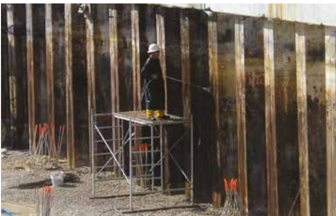
The interlocks of the piles were cleaned and seal-welded to render the excavation watertight
