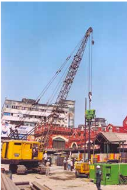
The sheet piles were installed with a resonance-free vibratory hammer
