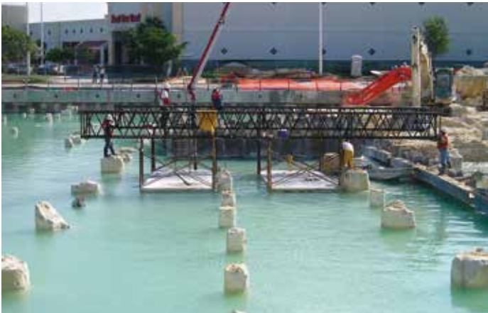
The underwater concrete of the bottom slab was poured with a tremie
