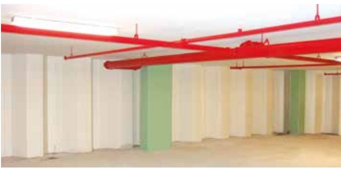
The coated sheet pile walls add an aesthetic aspect to the finished car park
