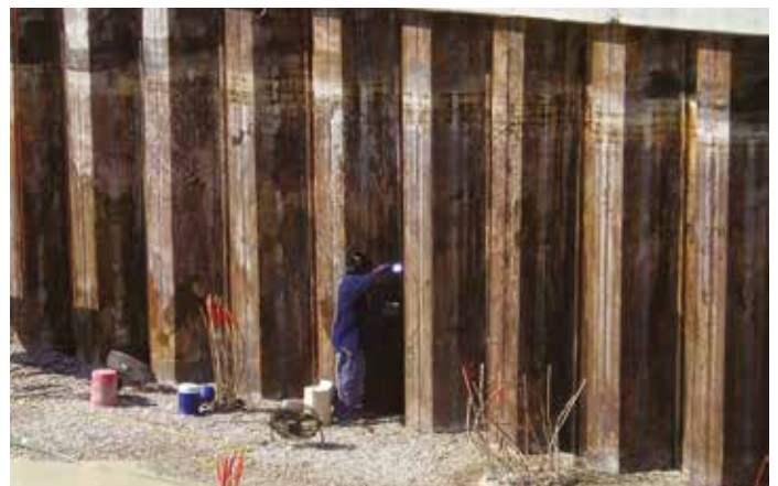
The interlocks of the piles were cleaned and seal-welded to render the excavation watertight
