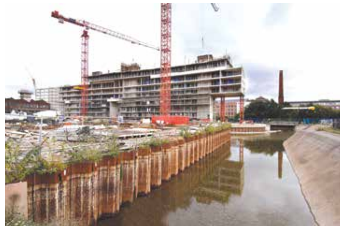
New canal arms were built in New Islington in 2003 using AZ 25 steel sheet piles as retaining elements
