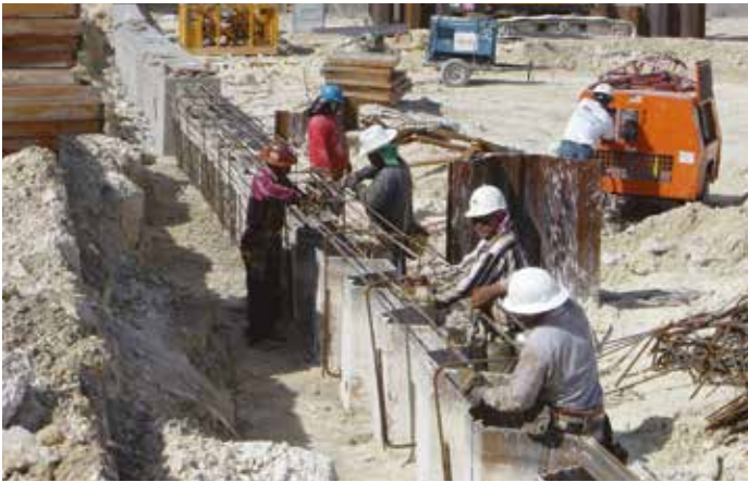
A capping beam incorporating temporary tie rods was placed at the head of the AZ 26 piles
