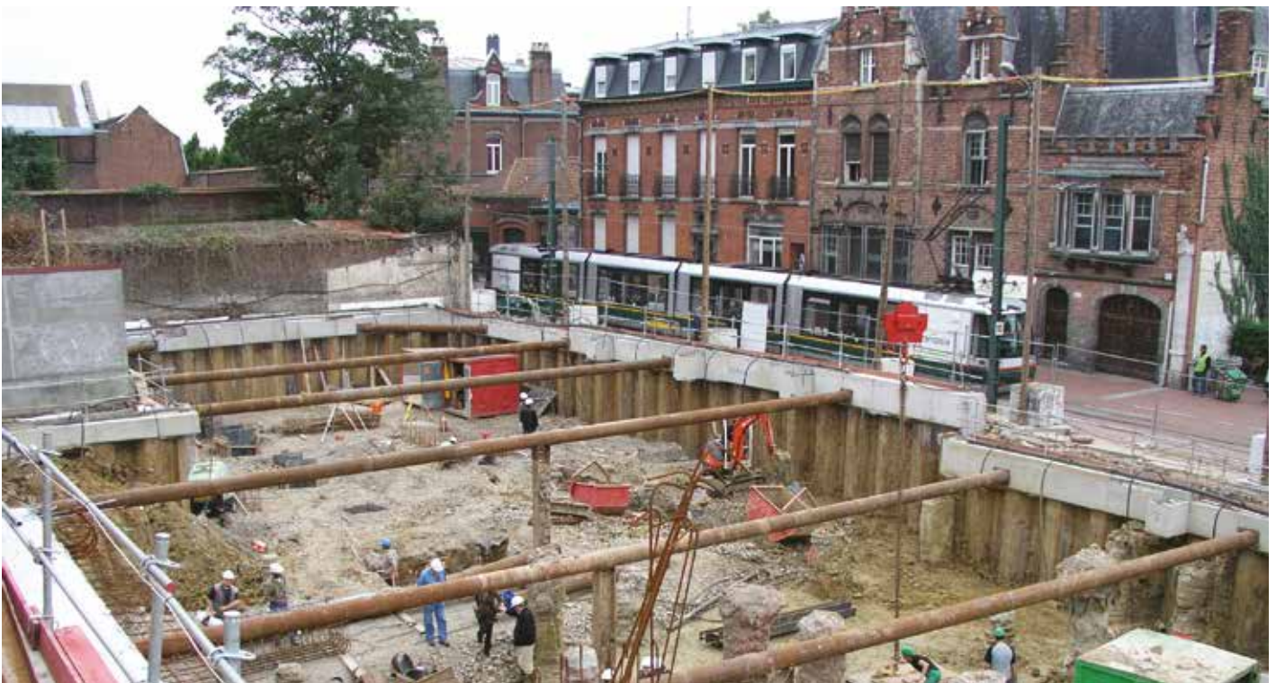
The underground car park beneath the residential building was built with a watertight sheet pile retaining wall
