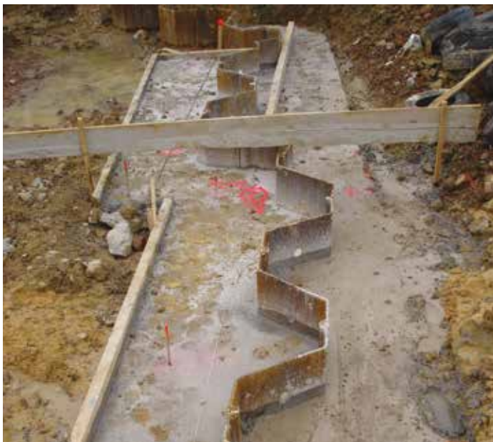
A concrete capping beam was then poured on to the head of the sheet piles
