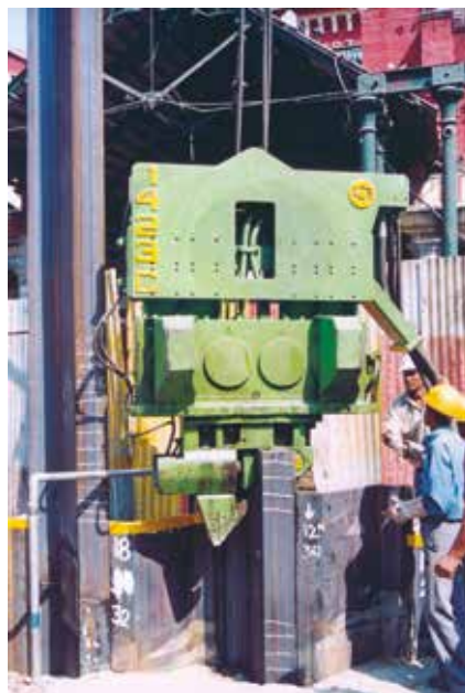
The sheet piles were installed with a resonance-free vibratory hammer
