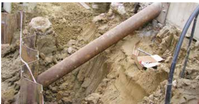
Horizontal reactions were carried by steel struts
