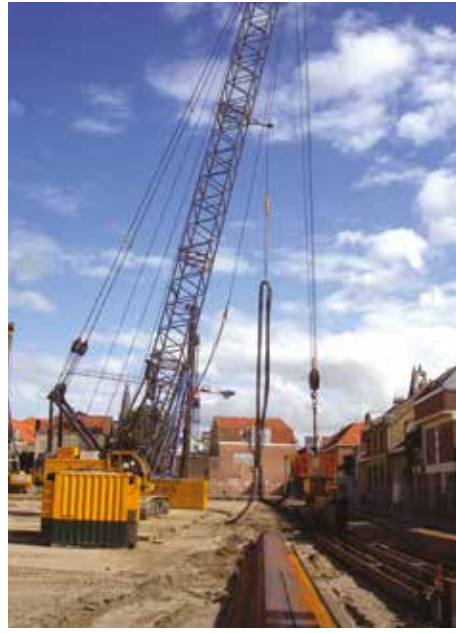
The AZ piles were installed with a PVE vibratory hammer with variable moment
