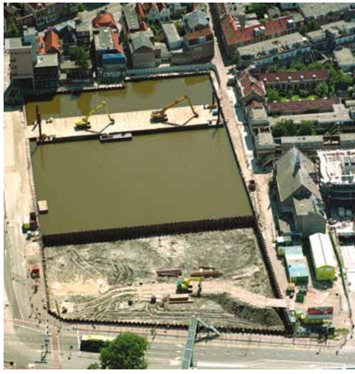
Car park P1 was built in two phases separated by a temporary AZ 36-700 sheet pile wall
