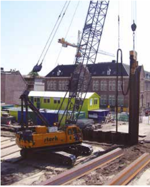
The contractor reduced noise and vibration emissions effectively by pre-drilling the soil before driving the sheet piles
