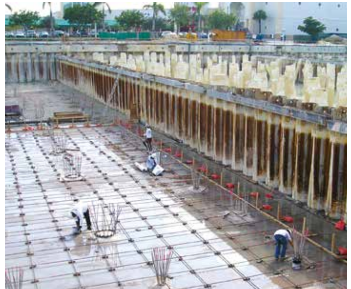
Temporary sheet piles separating different parts of the excavation were held together with walings
