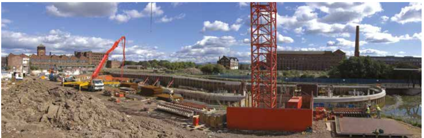
The soil and water retaining sheet pile walls enabled construction in the dry
