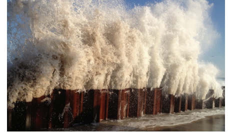
... to provide water containment, earth retention and excavation support.
