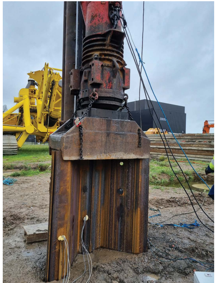
Driving the instrumented sheet pile A using a diesel Impact hammer (Phase 2)
