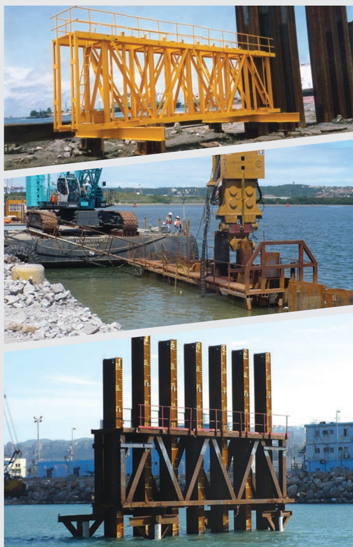
Fig. 16. Driving templates and their support.
