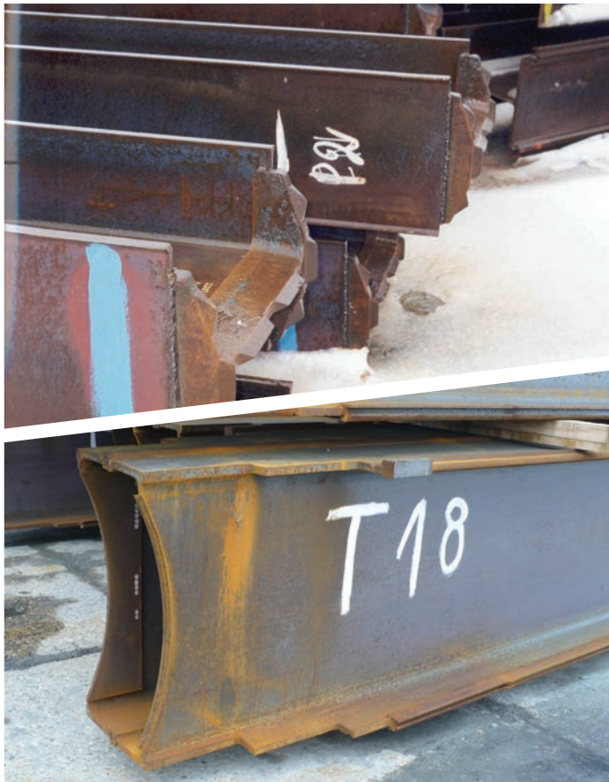
Fig. 24. Reinforcing of the tip of the pile with steel plates / shoes welded on the king pile toe.
