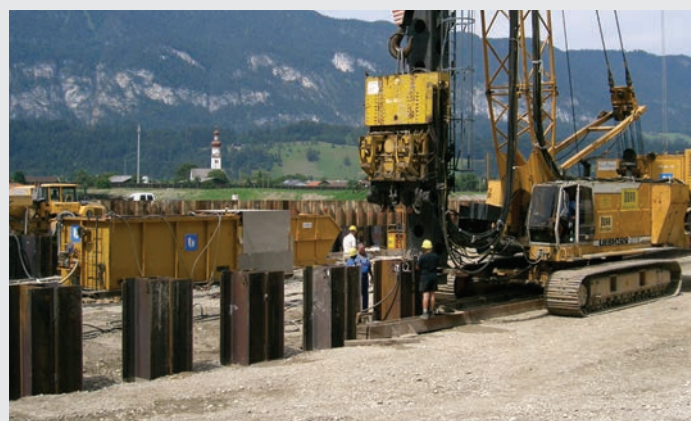
Fig. 18. Template with a single level and piling equipment guided on a fixed leader.
