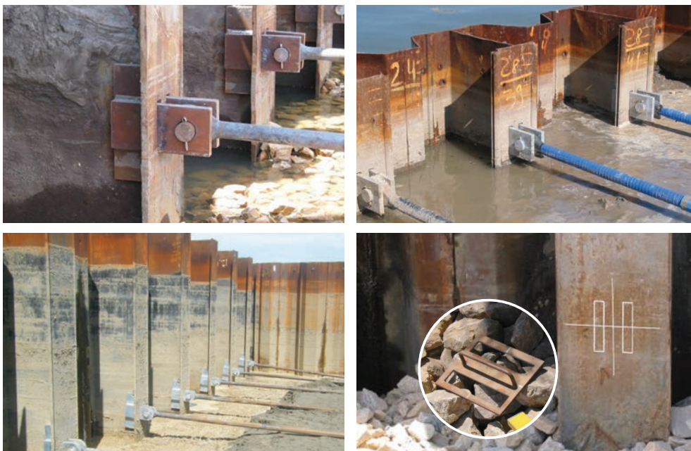
Fig. 27. Installation of the T-connectors at the job-site.
