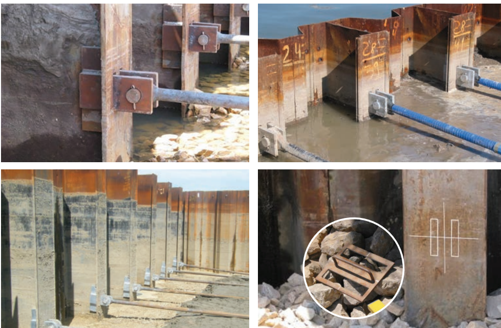
Fig. 27. Installation of the T-connectors at the job-site.
