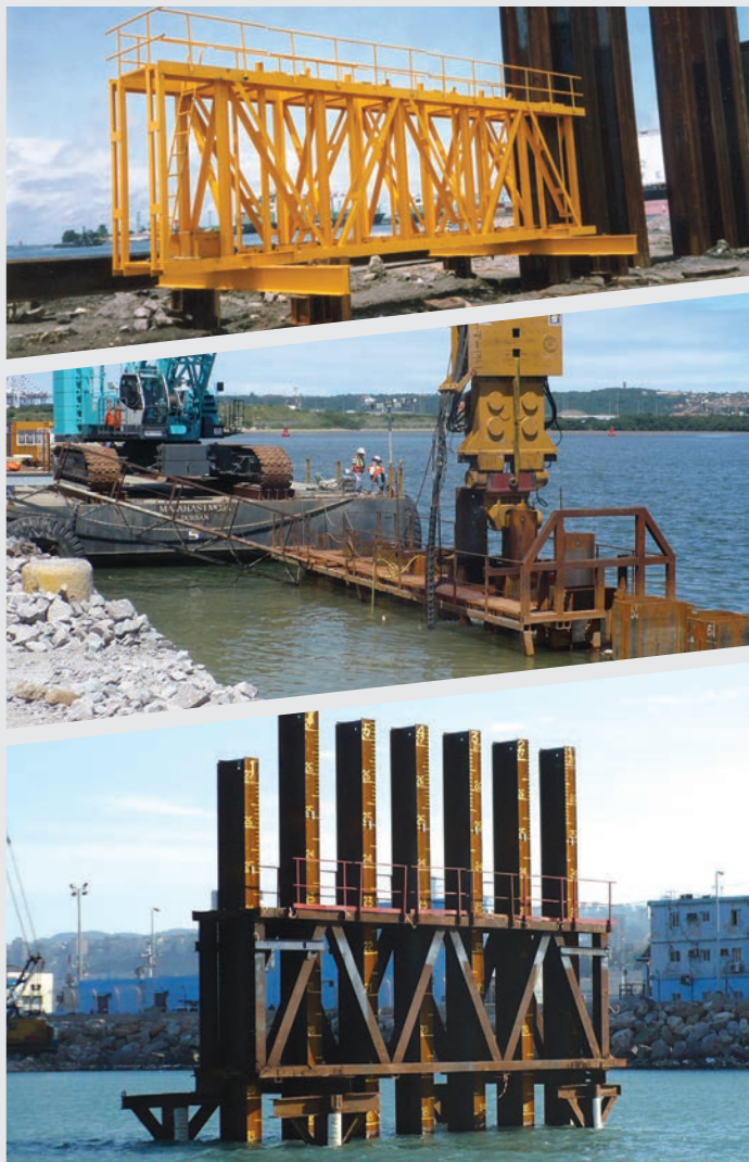
Fig. 16. Driving templates and their support.
