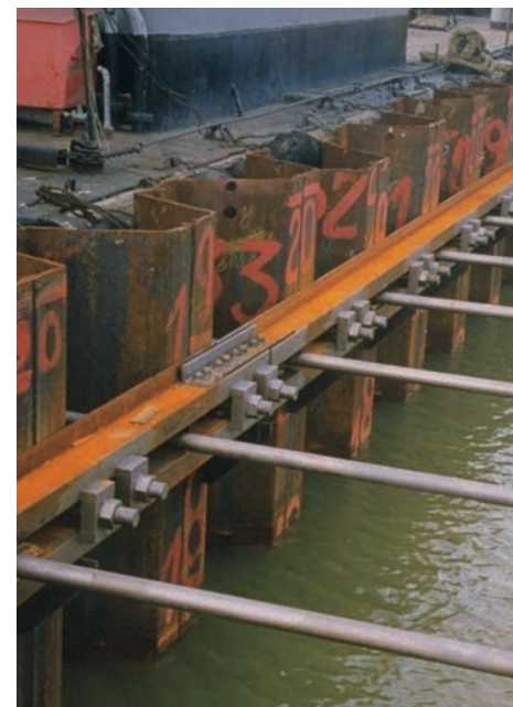
Fig. 28. Conventional anchor solution with tie-rods, walers,...
