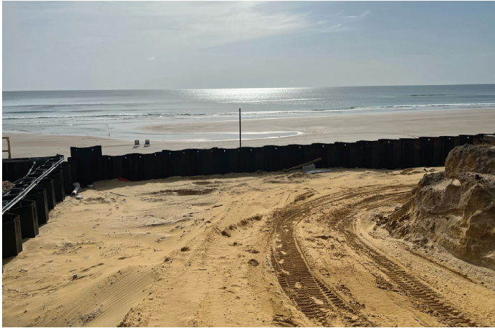
View of the jobsite
