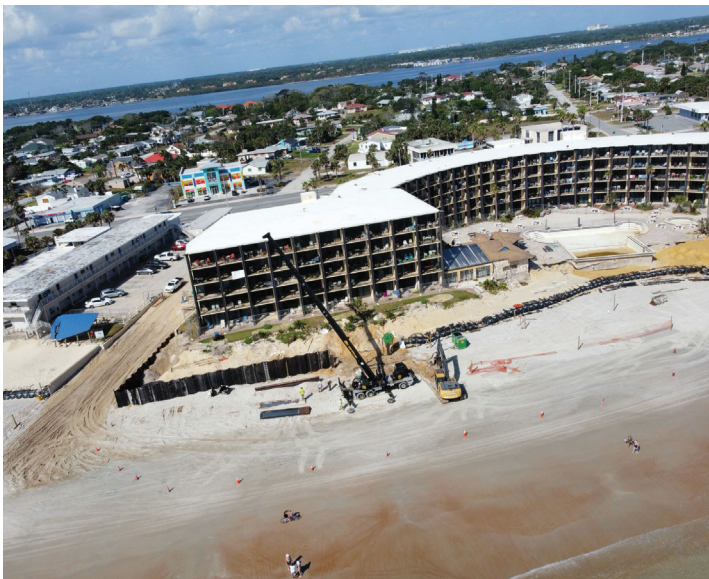
Aerial view of the jobsite
