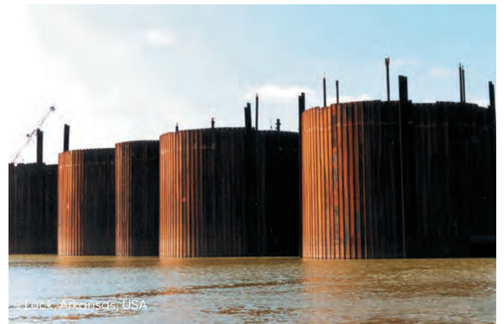
Diaphragm cells with 120^\circ junction piles.
