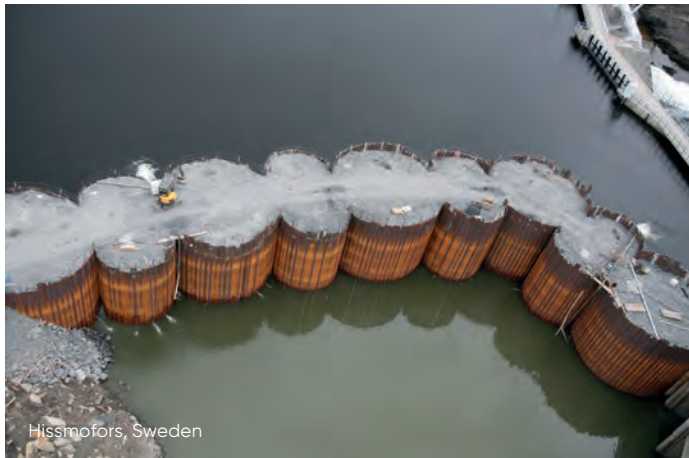
Circular cells with 35^\circ junction piles and one or two connecting arcs.
