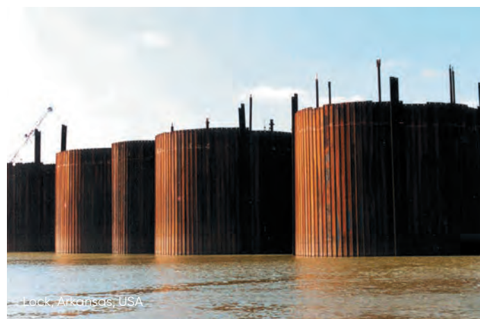
Diaphragm cells with 120^\circ junction piles.
