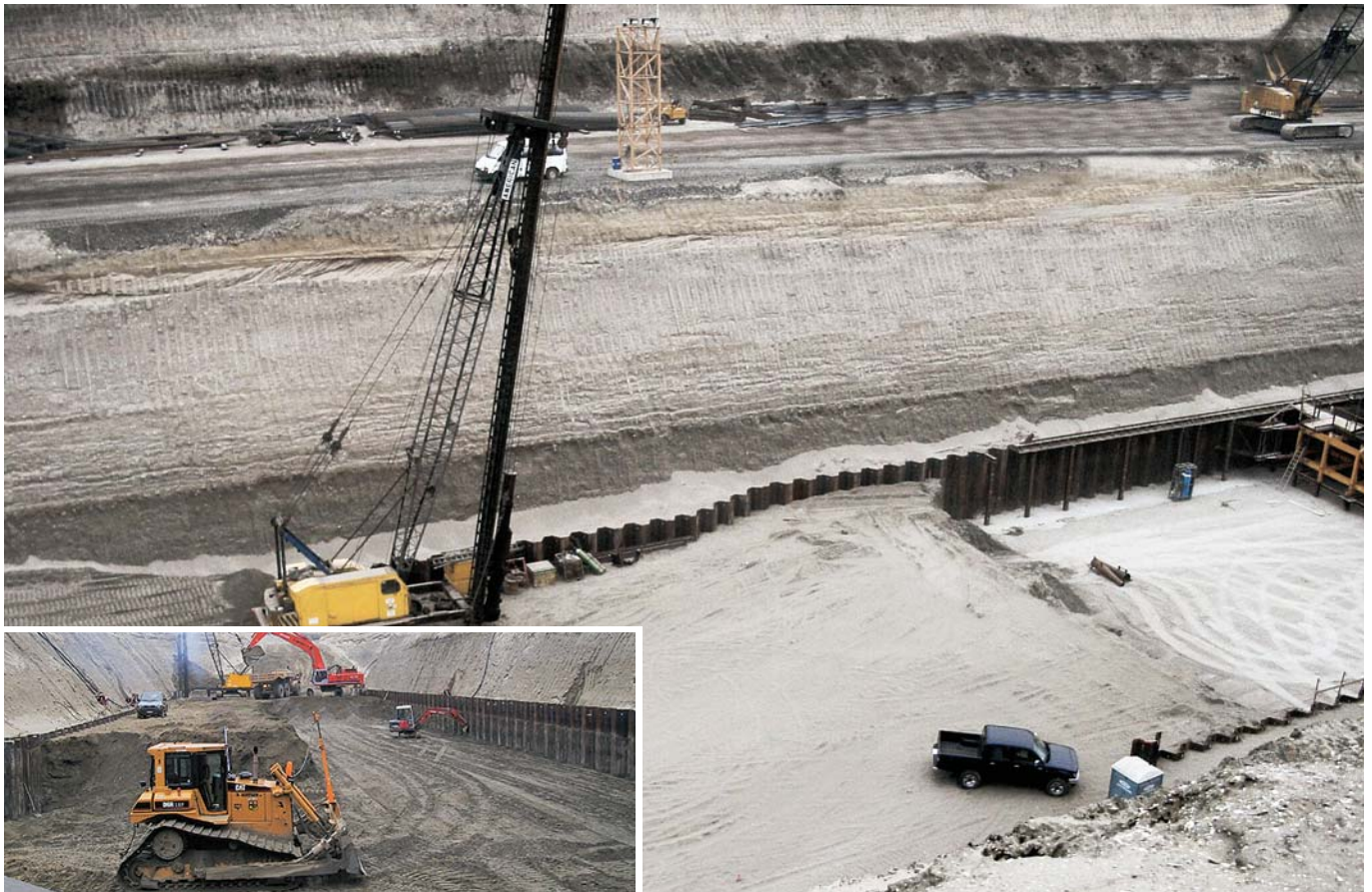
The AZ sheet piles were installed with a diesel hammer
