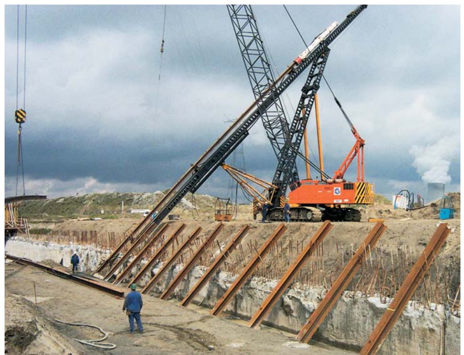
Steel MV piles take the tensile forces of the entrance walls
