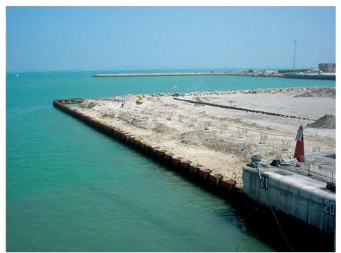
Once the sheet pile wall was installed, the area behind it was backfilled
