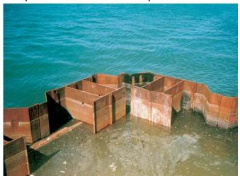
The wall's corner consists of AZ 18 piles that were also used as intermediary piles
