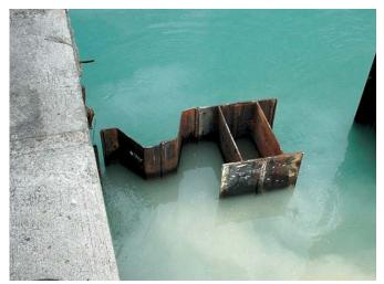
The connection between old and new quay consists of a steel plate welded to the first sheet pile
