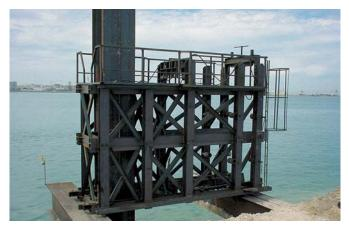
The driving template was placed on the embankment
