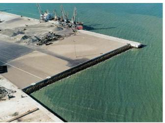
The quay extension required 1,600 metric tons of sheet piles
