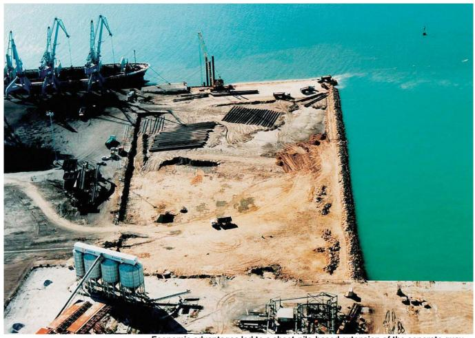
Economic advantages led to a sheet-pile-based extension of the concrete quay
