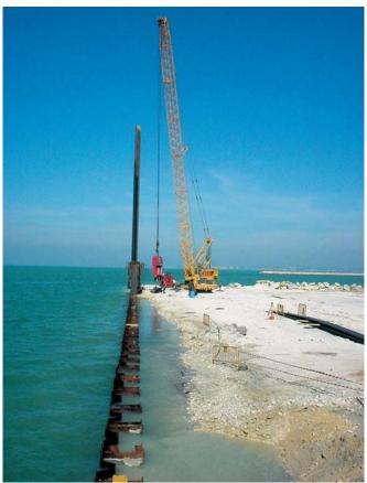
A berm of backfilled sand supported the driving equipment
