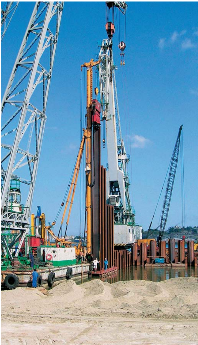
Several sheet piles were installed from a barge; others were driven with land-based equipment
