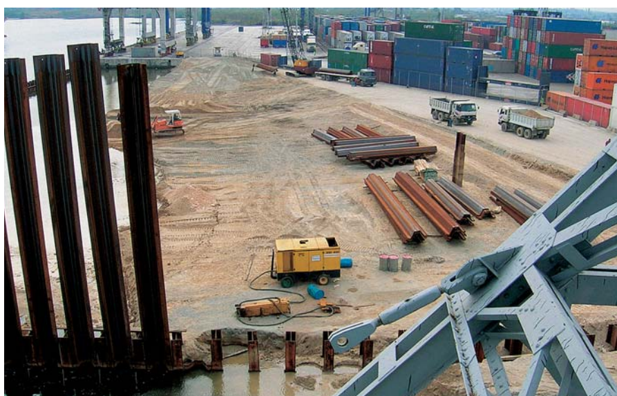
The AZ piles were inserted between the HZ piles then driven to design depth
