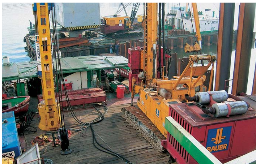
Bauer's pile-driving equipment: impact hammer and vibratory hammer
