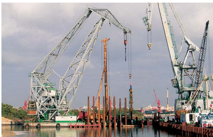
A locally hired floating crane assisted the installation of the combined sheet pile wall
