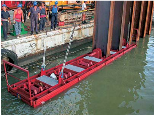
Precise positioning of the HZ king piles was guaranteed using a double-level template
