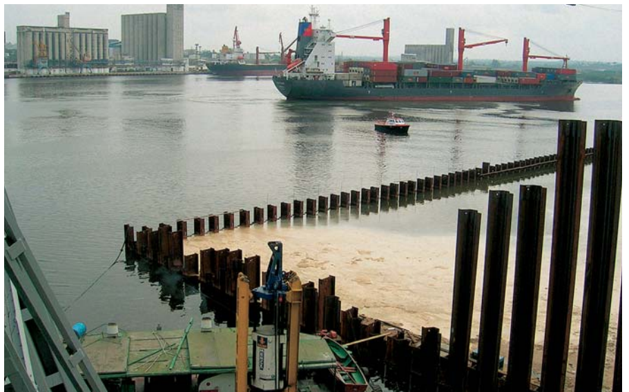
The area behind the quay wall was backfilled with dredged sand
