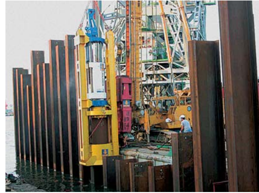
The HZ piles were driven by vibratory hammer until refusal, then taken down to design depth by impact driving
