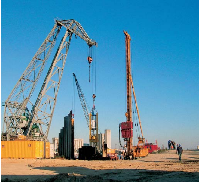
The HZ piles were driven by vibratory hammer until refusal, then taken down to design depth by impact driving
