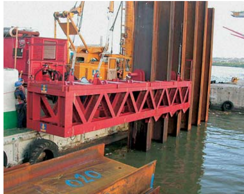
Precise positioning of the HZ king piles was guaranteed using a double-level template
