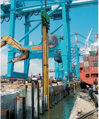
A special beam transmitted the vibration energy to the underwater AZ-piles
