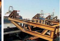
Neoprene shields attached to the template protected the coating system during installation
