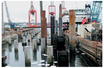
The steel sheet pile wall that stabilised the structure was installed from a barge
