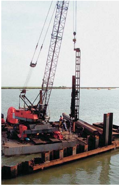
Delmag diesel impact hammer
