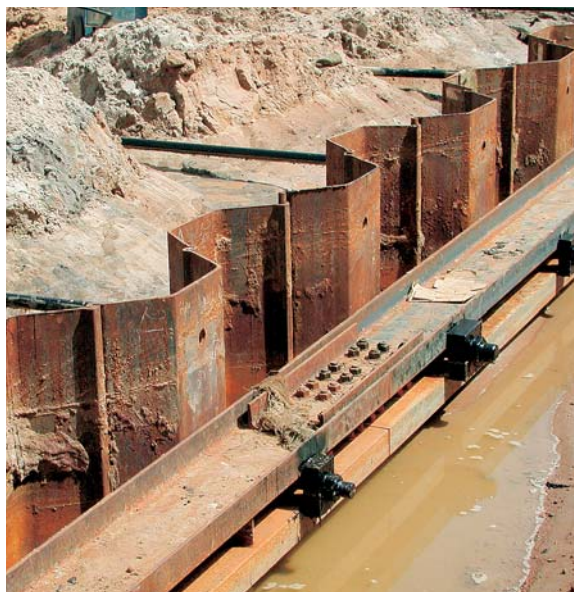
Anker Schroeder provided the entire tie-back system
