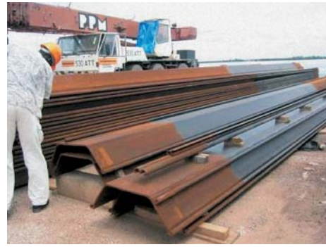
A three-layer coating system was applied to guarantee a long lifetime
