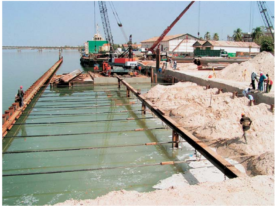
190 tie rods in different lengths were supplied by Anker Schroeder
