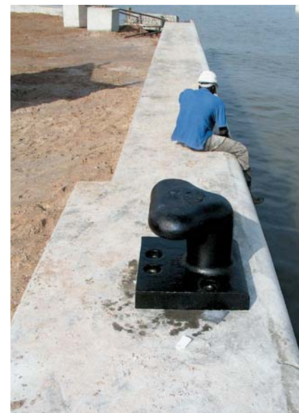
Finished quay with bollard system
