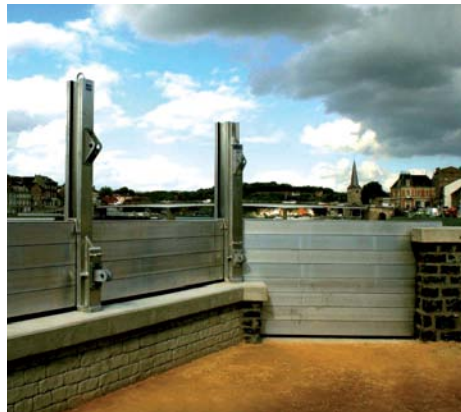
Demountable protection during assembly
