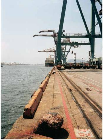
It was therefore decided to opt for a high-strength steel sheet pile solution to deepen the quays. The new underwater sheet pile wall was to be placed in front of the toe of the existing quay wall.
