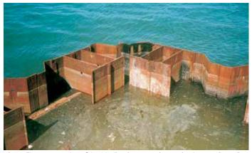
The wall's corner consists of AZ 18 piles that were also used as intermediary piles.
