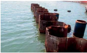
The 624-m sheet pile wall will enlarge the mooring area.
