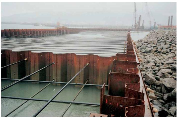
Numbers of tie rods cross over each other to connect the main and return walls to their respective anchor walls.
