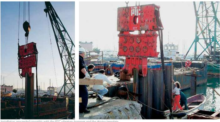
Installation proceeded smoothly with the PTC vibratory hammer and the driving template.
