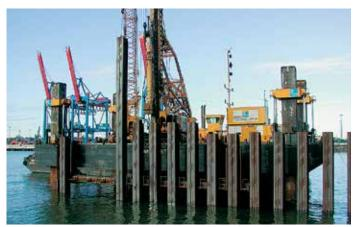
The steel sheet pile wall was installed with the help of a jack-up platform.
