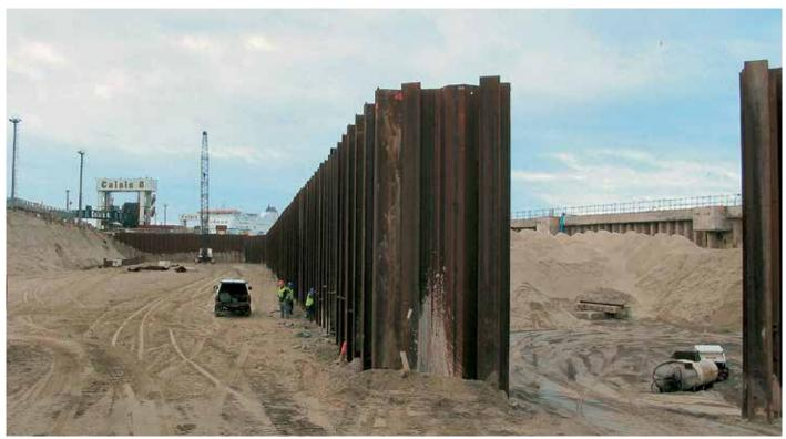
Bentonite and other filling materials prevented the possibility of the very fine sand washing out through the interlocks.
