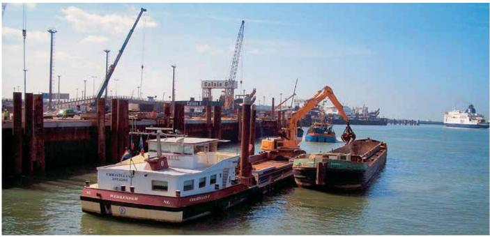
The rocks forming the old harbour bed were removed by a crane mounted on a barge.
