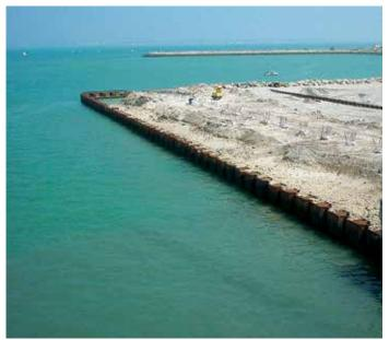
Once the sheet pile wall was installed, the area behind it was backfilled.
