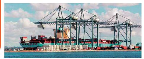
The new terminal will feature super-post-Panamax cranes and a water depth of 15.5 m.
