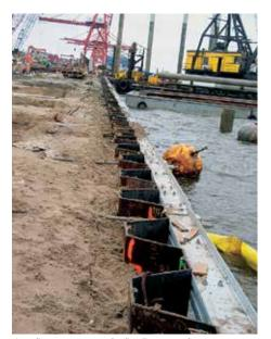
A waling system evenly distributes anchor forces into the sheet pile wall.
