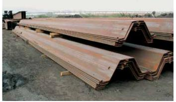
Wooden spacers prevent damage to the stored AZ piles.
