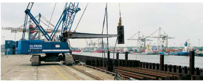
A crane lifted the preassembled anchors into position.
