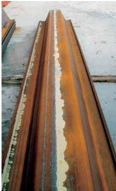
A sealing system, the waterswelling Roxan system, was inserted into the piles interlocks.
