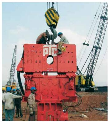
The contractor opted for the PTC 60HD heavy-duty vibratory hammer.
