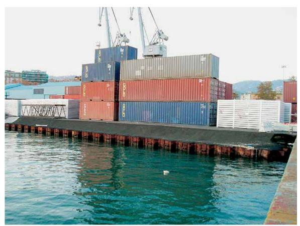
Thanks to the combined-wall system the new quay now offers a water depth of 10 m.
