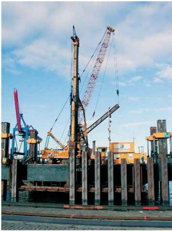
A crane lifted the sheet piles into the template.
