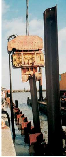
The vibratory hammer was the ideal tool to install the AZ intermediary sheet piles.
