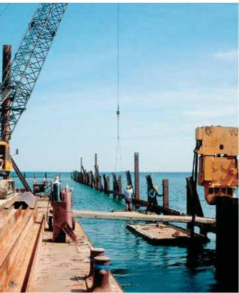
The crane, vibratory hammer and sheet piles were loaded on a barge.
