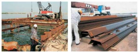
A three-layer coating system was applied to guarantee a long lifetime.
