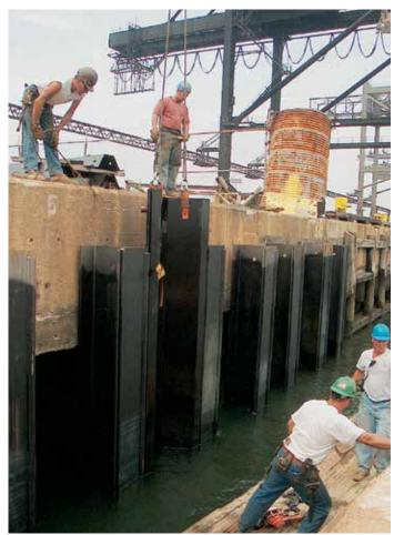
The heads of the HZ king piles remained above the water line, which facilited their installation...
