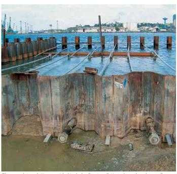
The complete solution provided includes front wall, tie rods, and anchor wall.
