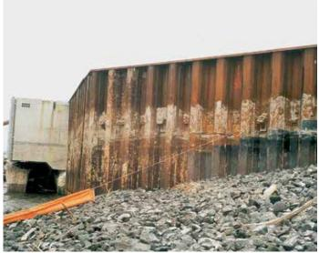
A sheet pile wall finishes off the terminal at both ends.
