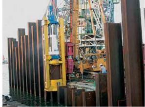
HZ piles were driven by vibratory hammer until refusal, then taken down to design depth by impact driving.
