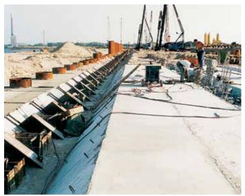
After pouring, the concrete of the relieving platform was covered with a 3.3 m sand layer.
