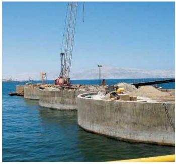
Concrete ring beams protect the cells.
