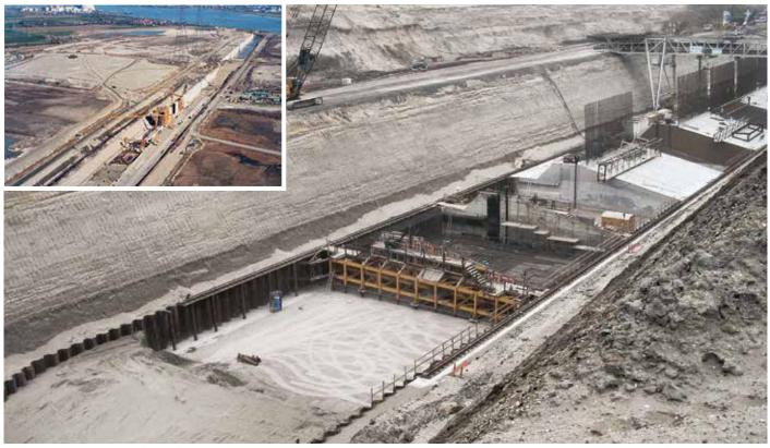
Over 6,000 t of steel sheet piles were used for the foundation of the quay walls.
