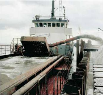
The cofferdam was filled with dredged sand.
