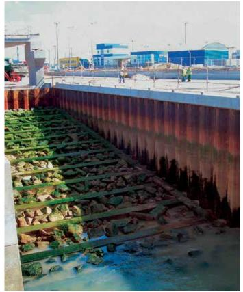
The 35 x 14 m sheet pile trench accommodates the lower access ramp.
