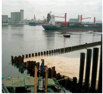
The area behind the quay wall was backfilled with dredged sand.
