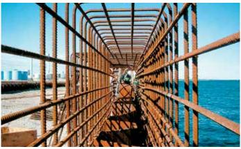
Reinforcement bars of the capping beam.
