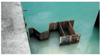
The connection between old and new quay consists of a steel plate welded to the first sheet pile.
