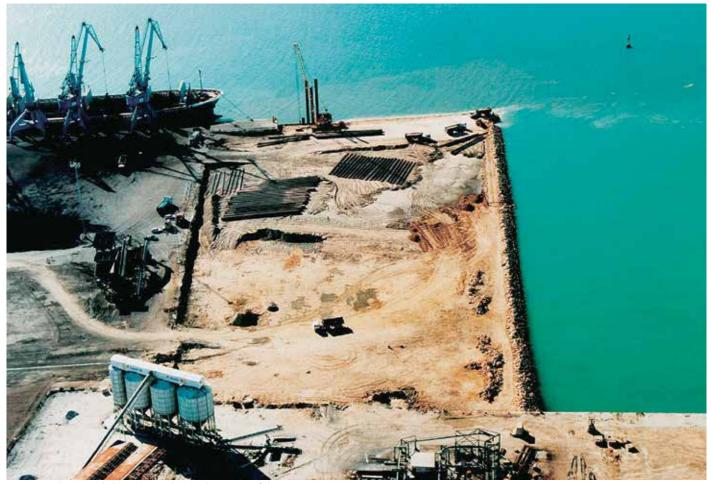
Economic advantages led to a sheet-pile-based extension of the concrete quay.
