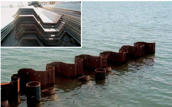
The structural system consisted of a sheet-pile soil-retaining wall, steel crane-foundation piles, and deflection-restricting batter piles.
