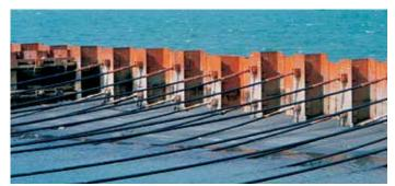
Two layers of tie rods connected main and anchor walls
