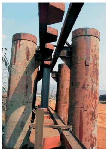
Two-level templates ensure correct horizontal and vertical positioning of the sheet piles.
