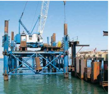
A jack-up barge and a template were used to install the HZ/AZ system.
