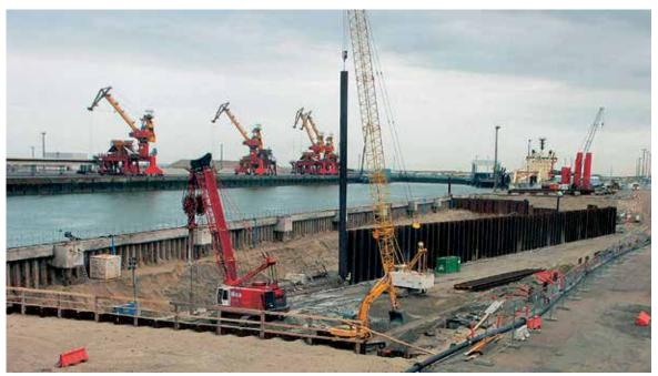
The old anchor wall had to be removed before the piles for the new Berth 9 were driven.
