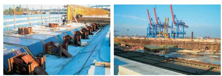
The load-relieving concrete superstructure installed at elevation +3 m provides for economical design of the combined sheet pile wall.
