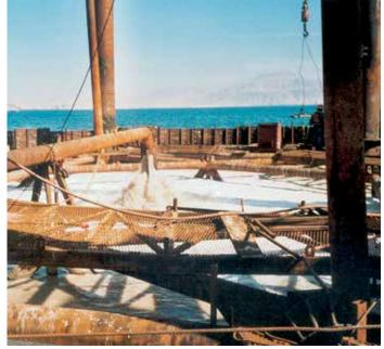
Sheet pile cells are usually filled with locally available sand.
