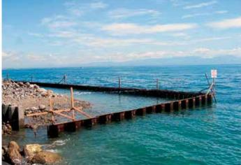
The new steel quay wall of Wharf 2 was placed 27 m ahead of the existing concrete wall.
