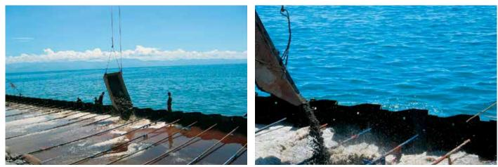
The area behind the AZ wall was backfilled carefully so as not to damage the tie rods.
