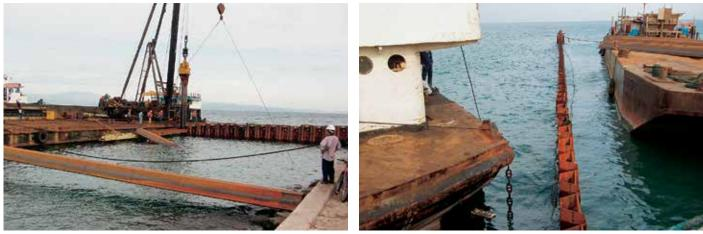
The two wharves were built using 380 AZ 34 double sheet piles as well as 80 AZ 26 double sheet piles.
