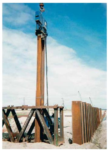
A two-level-template ensured straightness during installation.
