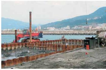
A large excavator was used to backfill the area between the main and anchor walls.
