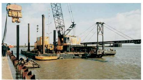
After installation of all the king piles, the AZ sheet piles were driven to El. - 20 m.
