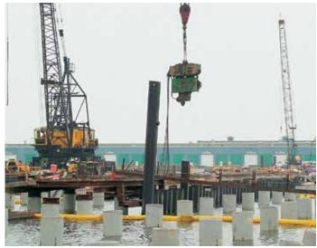
Installation of the basin's impervious sheet pile wall.
