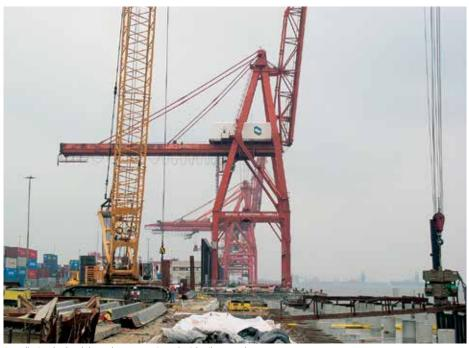
Installation by land-based crane equipped with vibratory hammer.
