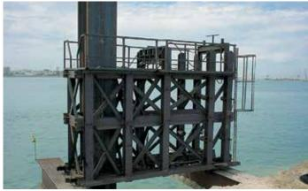
The driving template was placed on the embankment.
