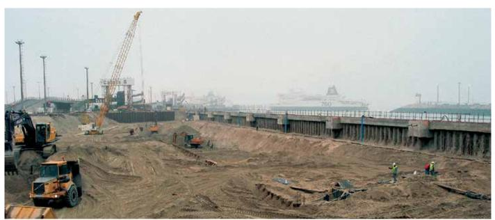
The existing PU 25 quay wall allowed the new wall to be driven in the dry.
