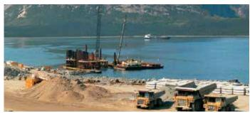
Piles were driven with barge-mounted equipment.
