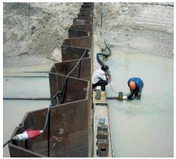
Tie rods were installed above the water line to facilitate the installation.
