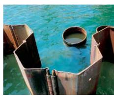
The special configuration of the AU 20 double piles led to a section modulus of 6,365 cm³/m.
