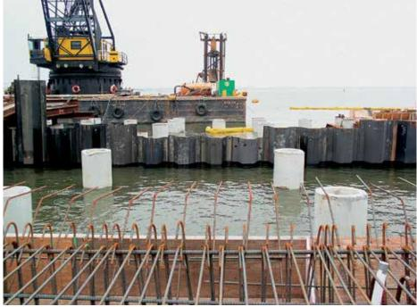
The AZ 36 sheet piles take the statical loads and act as an impervious water barrier.
