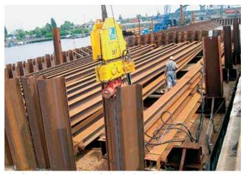
The vibratory hammer was attached to the sheet piles prior to installation of the anchors.
