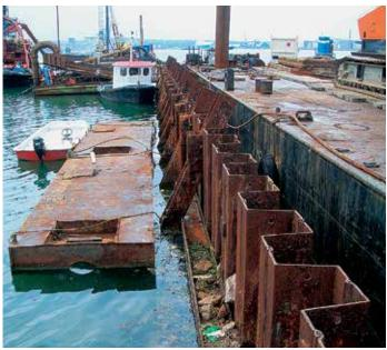
The new quay wall was temporarily fixed with inclined piles
