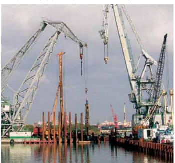
A locally hired floating crane assisted the installation of the combined sheet pile wall.
