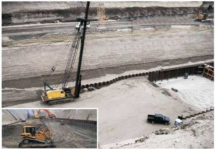
The AZ sheet piles were installed with a diesel hammer.
