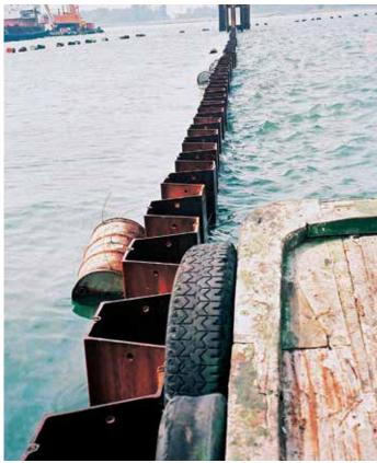
Great care was taken to achieve the exact design length of the quay wall. The contractor welded rebars on the inside of the AZ 46 sheet piles to prevent rotation of the middle interlock which could have increased or reduced the width of the AZ 46 double piles. The target wall length was achieved by driving the quay wall in an optically controlled straight line. The contractor relied on the help of a driving guide for installation of the greater part of the 330-m quay wall, however.
