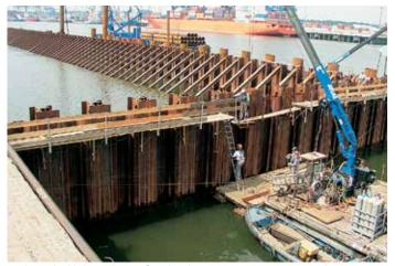
Each HZ double king pile was fitted with an HP 400 x 122 tension pile.
