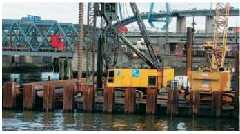
Because of the extreme soil conditions, pre-drilling was necessary to facilitate installation of the AZ piles.
