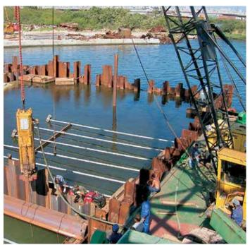
Driving of steel sheet piles with barge-mounted equipment.
