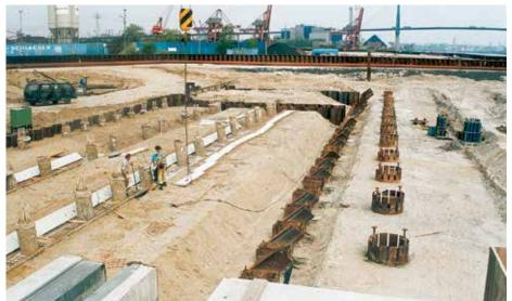
The low-level superstructure slab is placed on top of the two sheet pile walls, steel tension piles, fender tubes & concrete piles.
