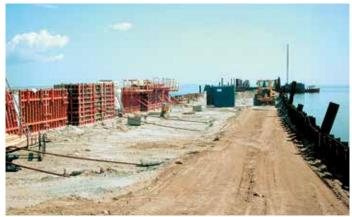
Formwork for the concrete capping beam.
