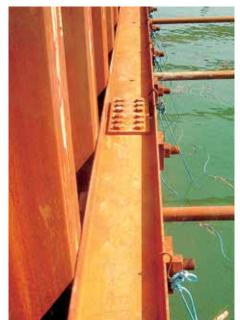
Horizontal beams were used as a driving template.
