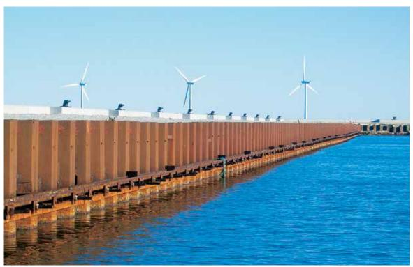
The sheet pile cofferdam forms an impervious barrier for the contaminated soil.
