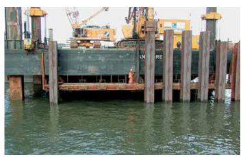
A template guides the head of the double HZ king piles.
