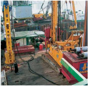
Bauer's pile-driving equipment: impact hammer and vibratory hammer.
