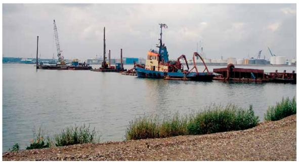
The construction equipment was mounted on barges to build the quay wall
