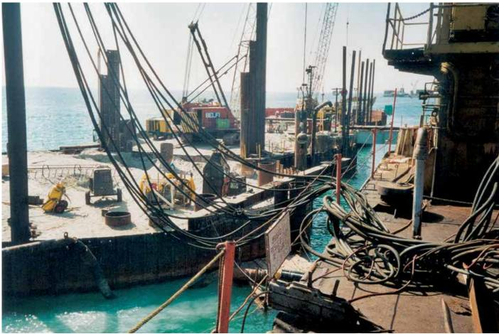
The filled cells are capable of supporting the construction plant.
