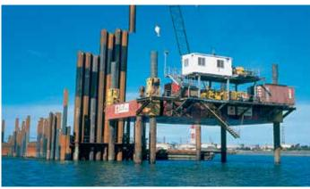
The main retaining wall was driven from a Flexifloat S-70 jack-up barge.
