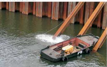
At an angle of 32°, the vibratory hammer was switched on to securely position the anchor.
