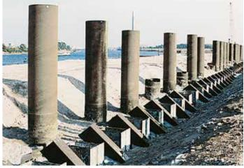
Tubes placed in front of the sheet pile wall act as fenders.
