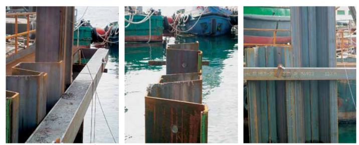
A template was used for the installation of the AZ piles.
