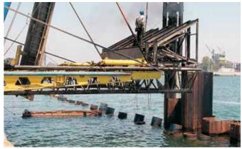
The contractor's template features two steel-tube guiding levels fitted with rubber fenders.
