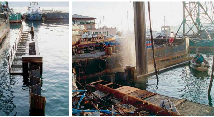
2,600 t of 24-m AZ 36 and 8-m AZ 18 sheet piles were installed.
