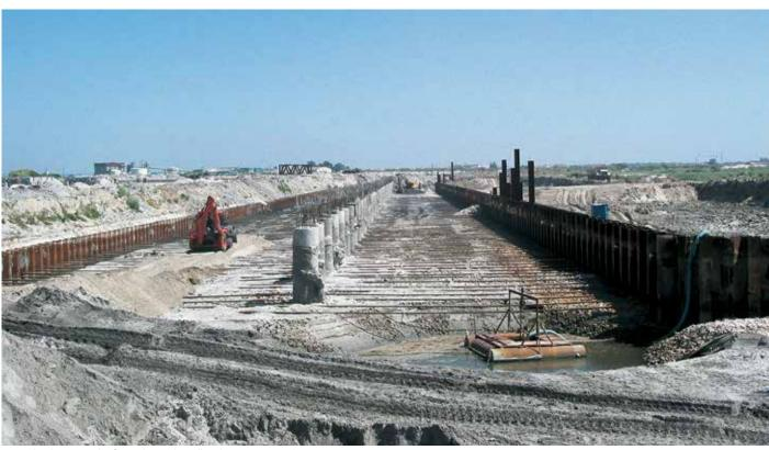
Crane loads rest on the front sheet pile wall and on concrete columns
