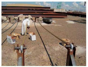
Corrosion-protection tape was wrapped around the anchors.
