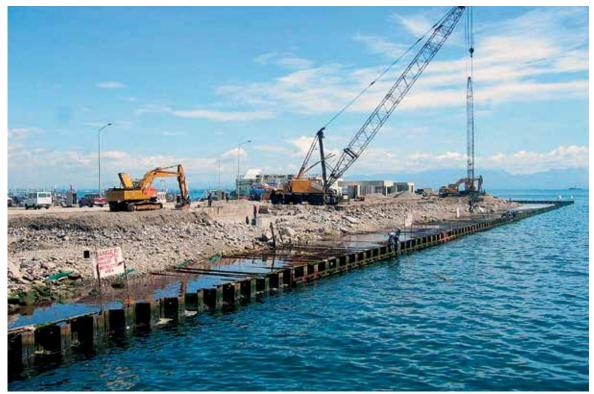
Two AZ sheet pile quay walls were required by the growing tuna fishing industry.
