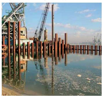
Driving of HZ king piles at the corner of the L-shaped wall.
