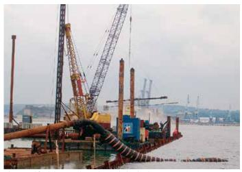
The crane lifted the tie rod together with the deadmen into position at a depth of eleven metres. Sand was pumped from a dredger to refill the area behind the sheet pile wall.
