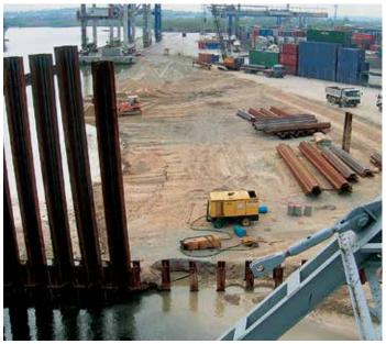
The AZ piles were inserted between the HZ piles then driven to design depth.
