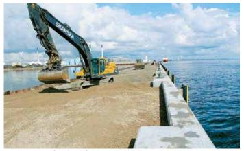
A capping beam fitted with fenders and bollards was placed on top of the sheet piles to finish off the construction.
