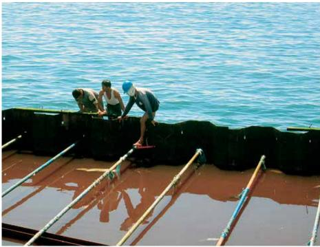
The tie rods consisted of several parts suitable for transportation in 40-foot containers.
