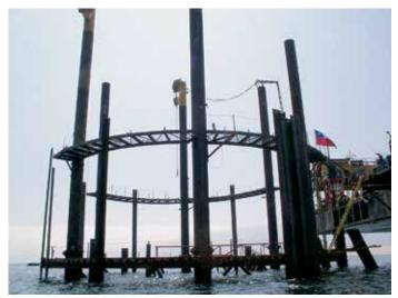
The breakwater is composed of eight cells with a diameter of 24 m.
