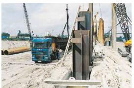
Due to difficult soil conditions, and as a means of reducing vibration, the sheet piles where driven in a bentonite-supported trench.
