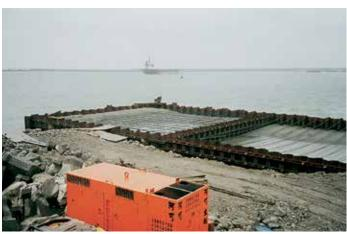
The 27.4-m return wall of Quay 15 consists of a combined wall with 14 HZ king piles.
