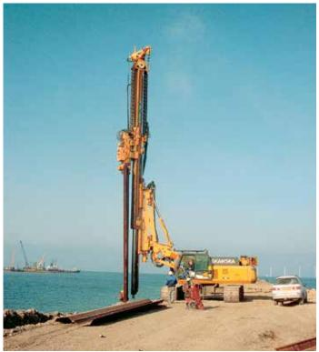
The PU 8 piles were driven into a berm by an excavator-mounted vibratory hammer.
