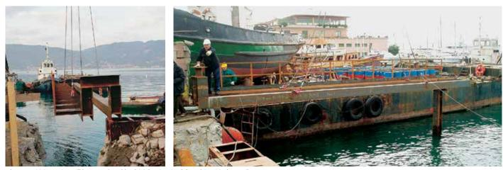
The new 400-m pier will be completed by 2006 using AZ 36 and AZ 18 sheet piles
