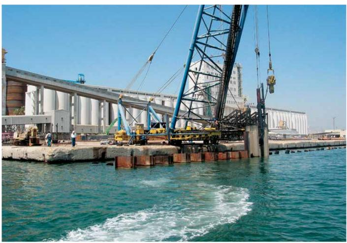
The existing concrete structure was modernised with the help of a jagged sheet pile wall.
