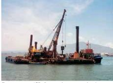
Two cranes, an ICE vibratory hammer and an impact hammer made up the installation equipment.
