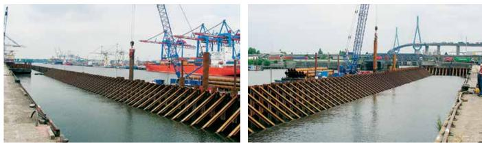
The new sheet pile wall of Berth 1 was placed 36.9 m in front of the old quay wall.
