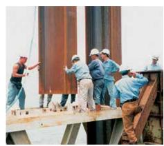
A two-level rigid template ensured the verticality of the king piles.
