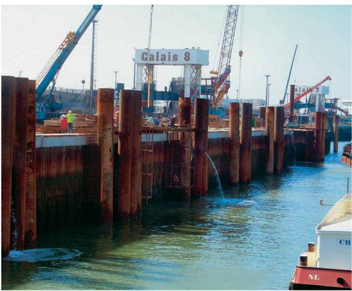
The steel tubes driven in front of the quay wall act as fenders.
