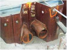
A hole was cut into the piles to pass the rebar tie rods.
