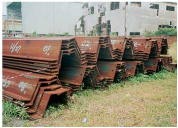
The deep excavation and seismic loads called for heavy-duty AZ 48 piles.
