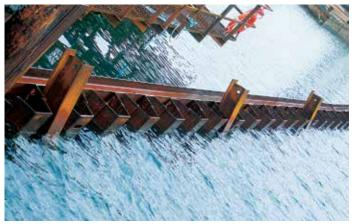
A steel beam was fixed to the main wall as waling.
