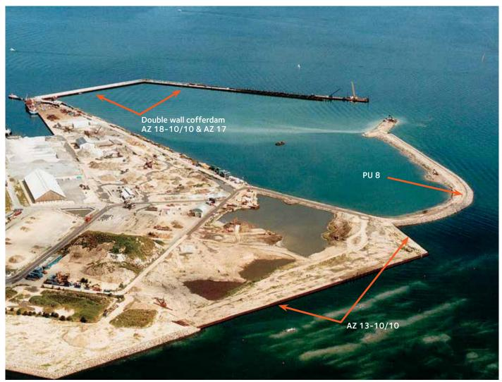
Different types of steel sheet piles were used for the cofferdam that functioned as a soil enclosure and harbour wall.
