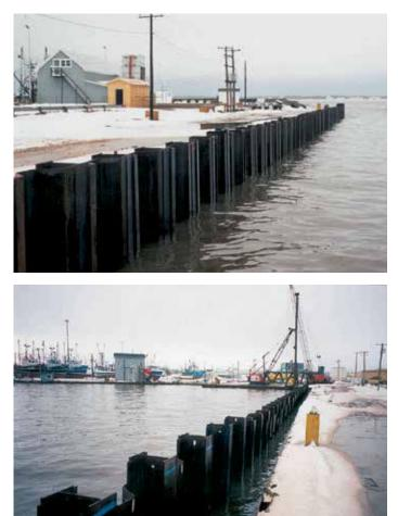
New sheet pile wall installed 1.5 m in front of the existing wall.
