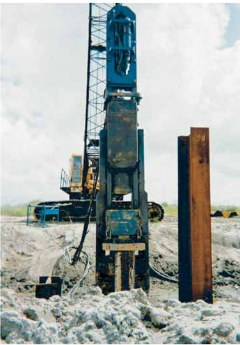
Due to the template the space between the king piles precisely fits one AZ pile.
