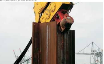
Two slots prevented jamming of the vibratory hammer.
