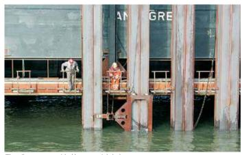
The pile toe was guided by a special sledge.
