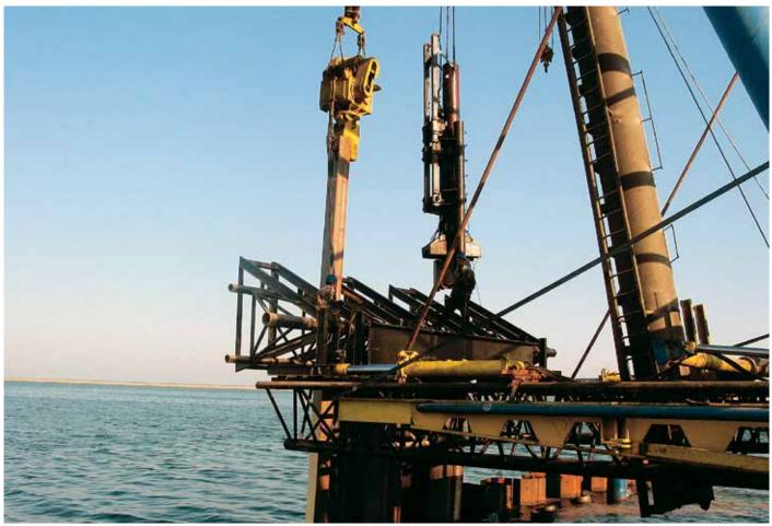
Both the vibratory and the impact hammer were mounted on the specially designed rail-mounted rig.
