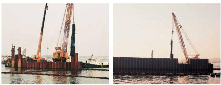
The sheet piles were installed in open water using barge-mounted vibratory and impact hammers.
