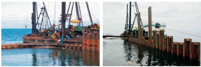
AZ double piles up to 21.5 m long were installed with barge-based driving equipment.
