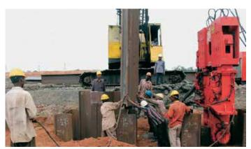
Due to the presence of weathered rock an impact hammer was needed to fully drive the sheet piles.
