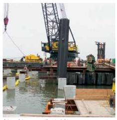
A template ensures the straightness of the sheet pile walls.
