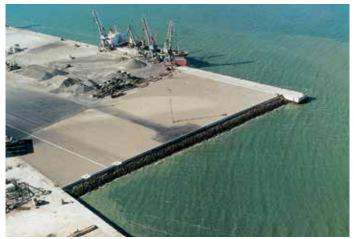
The quay extension required 1,600 metric tons of sheet piles.
