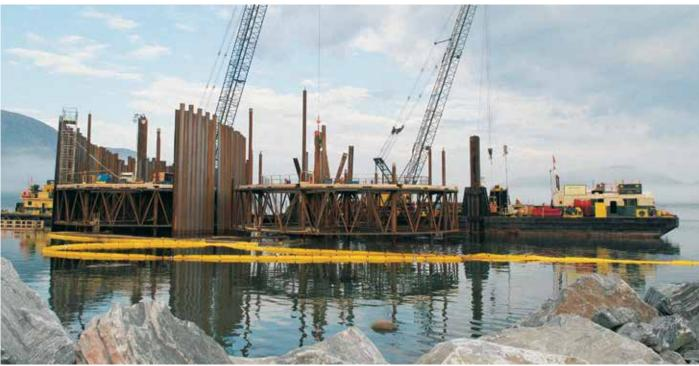
The sheet piles were installed with the help of a template.
