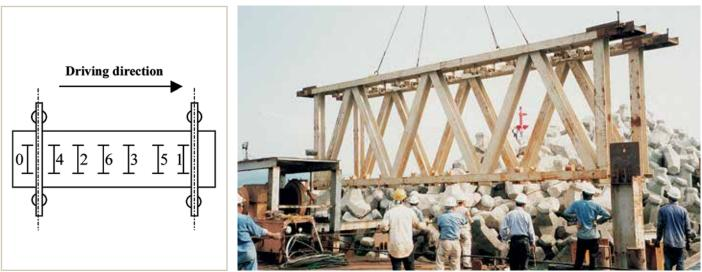
The "Pilgrim Step" driving sequence ensures that the piles encounter uniformly compacted soil during installation.
