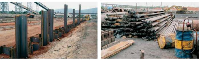
The Indian designer Howe opted for an anchored HZ/AZ combined sheet pile quay wall.
