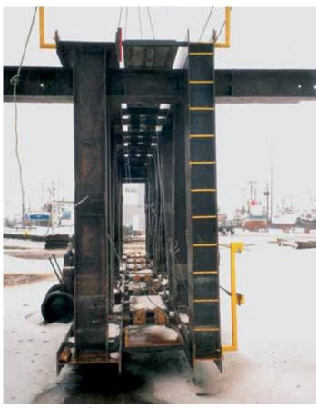
Eight guiding shoes - four per template level - guide each HZ king pile.
