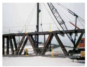
The two-level template ensures the king piles are correctly positioned for driving.
