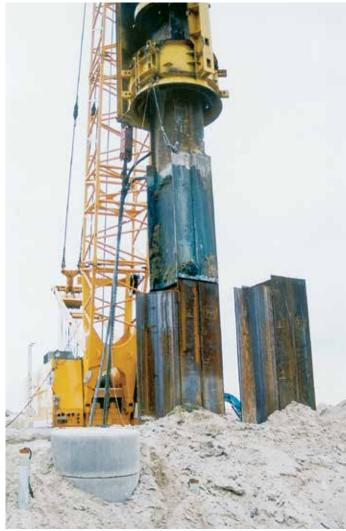
The heavy sheet pile elements were driven to a depth of 30.5 m with an impact hammer.
