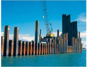
The project's design lifetime of 50 years called for two layers of tar-free epoxy coating.
