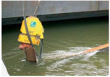
The entire anchorage system was lowered to the harbour bed with the vibratory hammer.
