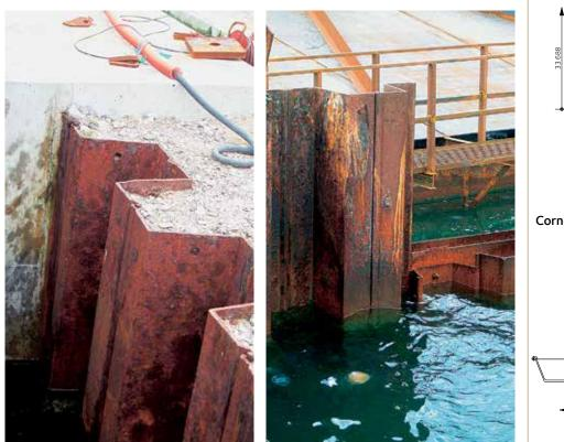
Detail A: End of capping beam of the old CT East. The existing sheet piles of CT East continued a few metres beyond the capping beam.
