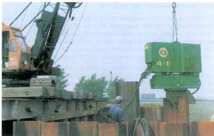
Figure 3.2.3-2: VIBRATEUR SUSPENDU
