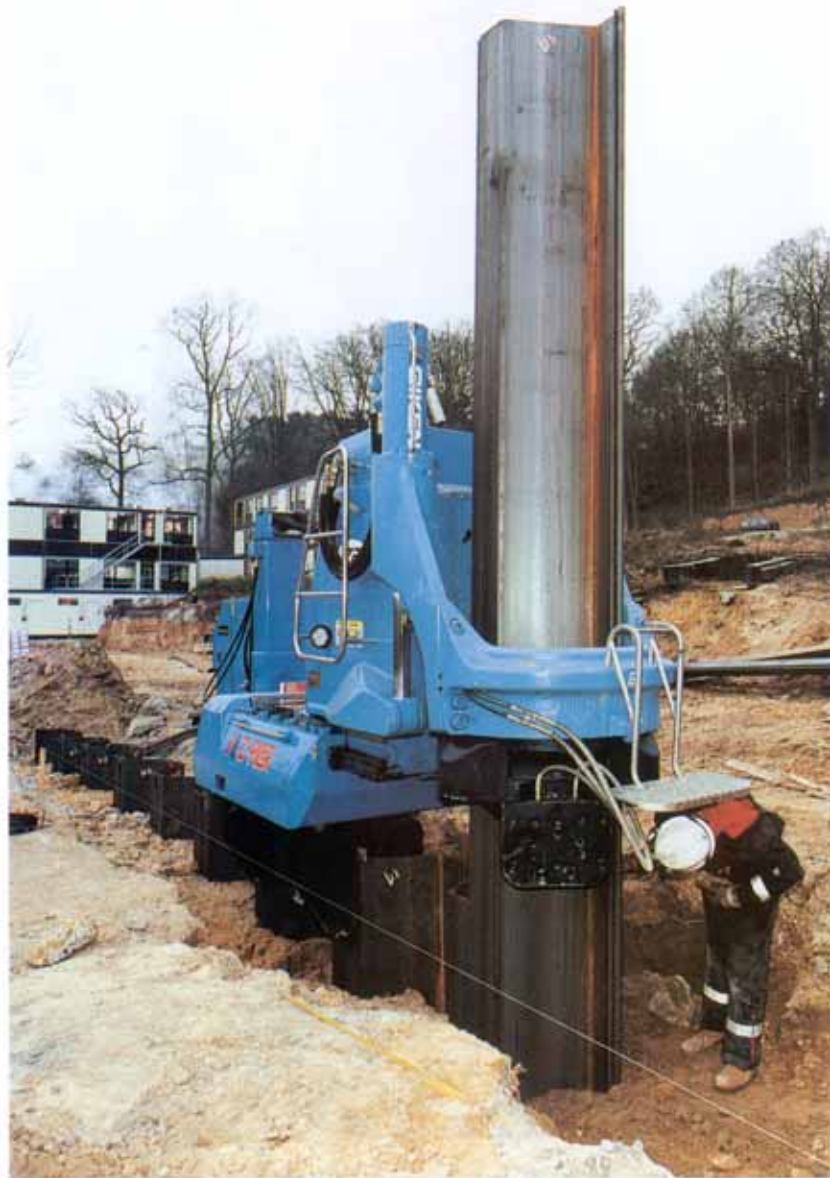
Figure 3.7-3: PRESSE HYDRAULIQUE (Type 3)
