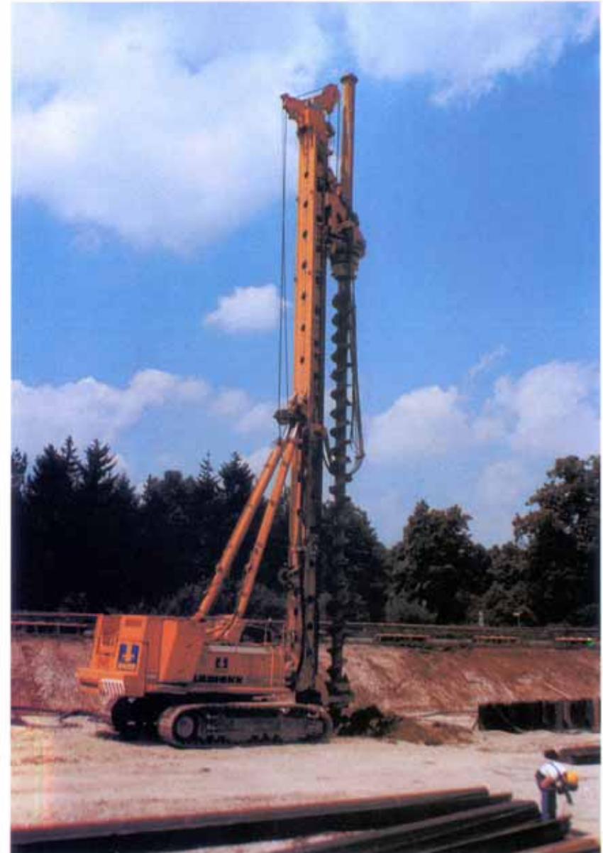
Figure 8.3: INSTALLATION DE FORAGE
