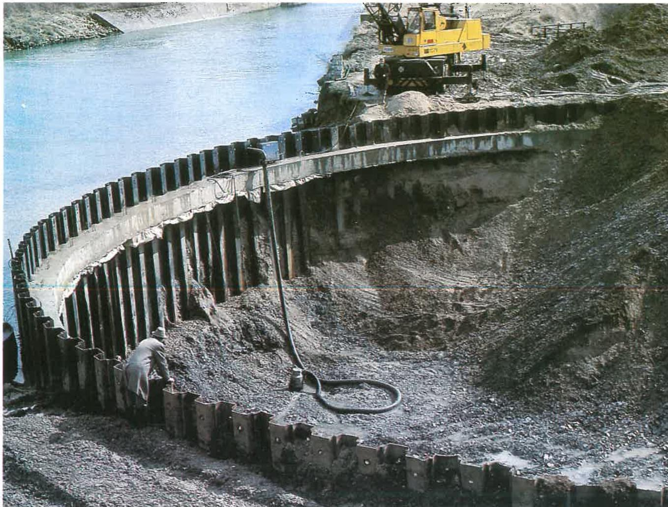
The increased size of pushed barge trains required the construction of a new guard gate. So as not to suspend navigation for any length of time the gate was constructed in the dry inside a circular cofferdam the main part of which was located on the bank ; the gate was then floated into position within a very short time span.
