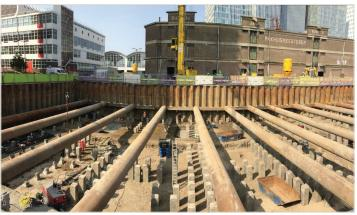
Figure 3.2. Excavation in sheet piles, parking facility Boston & Seattle, Rotterdam, The Netherlands. Courtesy of KÖCO.
