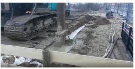
Figure 3.11. SoilMix wall in execution in vicinity of active railway, station Blerick, the Netherlands.
