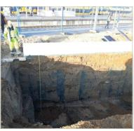
Figure 3.13. SoilMix wall excavated in vicinity of active railway, station Blerick, the Netherlands.
