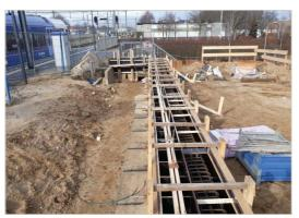
Figure 3.12. Capping beam on top of SoilMix wall in vicinity of active railway, station Blerick, the Netherlands.
