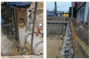
Figure 3.15. Secant pile wall, installation (left) and excavation (right), https://www.vsf.nl/nl/funderingen/wanden/boorpalenwanden.
