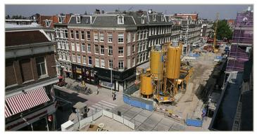
Figure 3.7. Fluid treatment plant, bentonite and cement silo's at inner-city project North South Line Amsterdam, the Netherlands.
