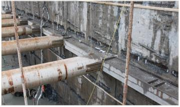
Figure 3.6. Connection with concrete deck and struts during excavation, project Garenmarkt, Leiden, the Netherlands.
