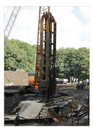
Figure 3.5. D-Wall grab with sled and elevated bentonite level, test site Noord Kasteel, Antwerp, Belgium.
