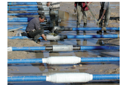
Site wrapping of connections
