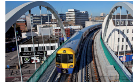
ASDO Structural Architectural tie bars
