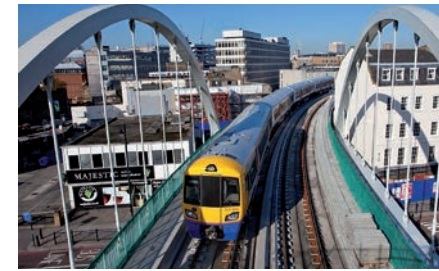
ASDO Structural Architectural tie bars
