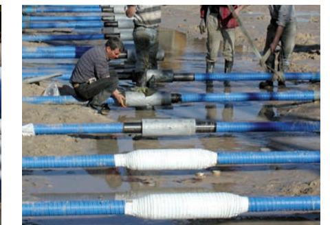
Site wrapping of connections
