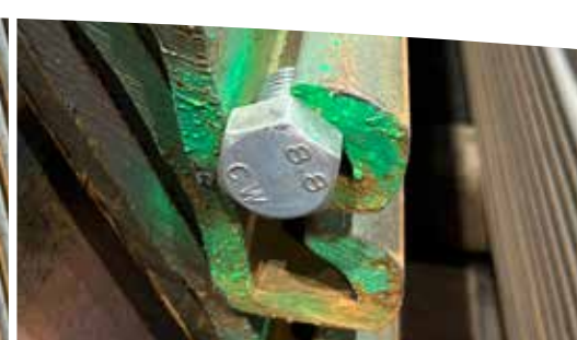
Bolt inserted in leading interlock.
