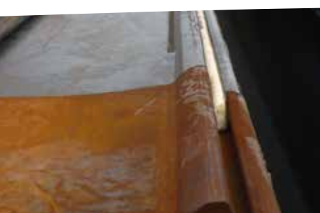
Closing interlocks with foam, grease or BeltanPlus.
