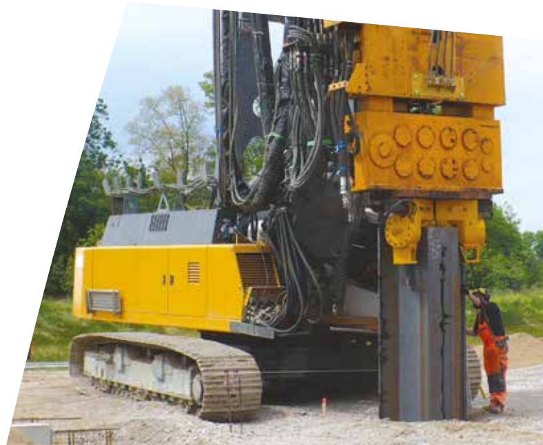
Leader-mounted vibratory hammer with double clamps.
